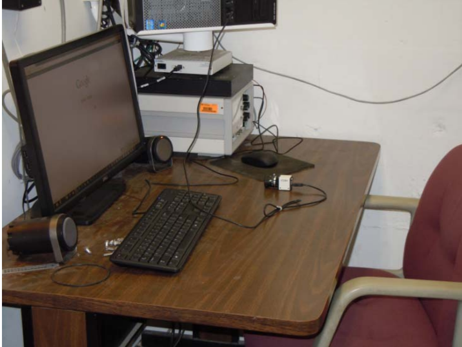
Figure A-11. SERF control room
