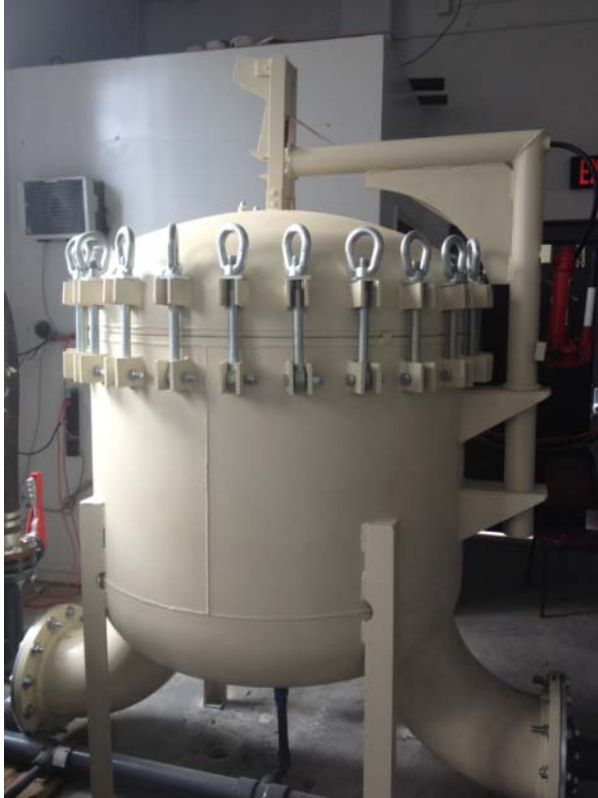
Figure A-13. Large-capacity filter
