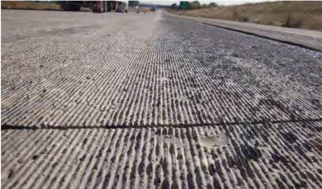
Figure 22. Roadway surface after conventional grinding.
