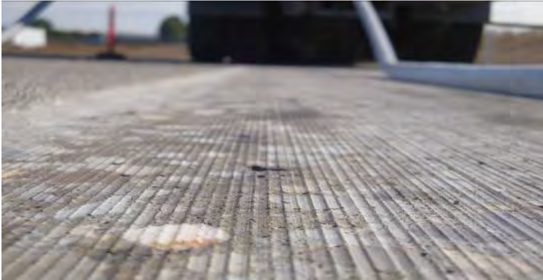
Figure 24. Pavement surface after fine grinding.
