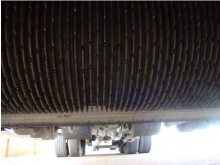
Figure 8. Grinding head for cutting the grooves on the second pass.
