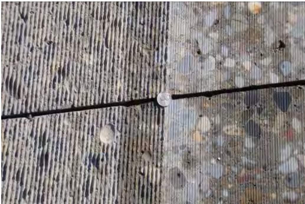
Figure 9. Conventional diamond ground surface on the left, fine flush grind surface of the NGCS first pass operation on the right.
