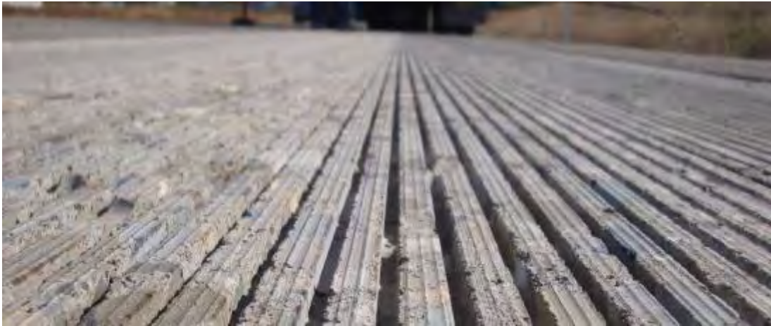
Figure 26. Pavement surface after tall blade grinding.
