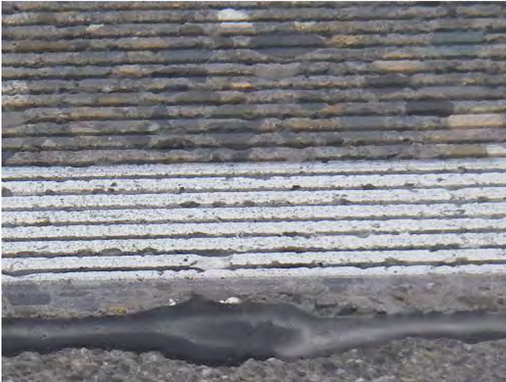
Figure 13. Close-up of NGCS with shoulder stripe in the foreground.
