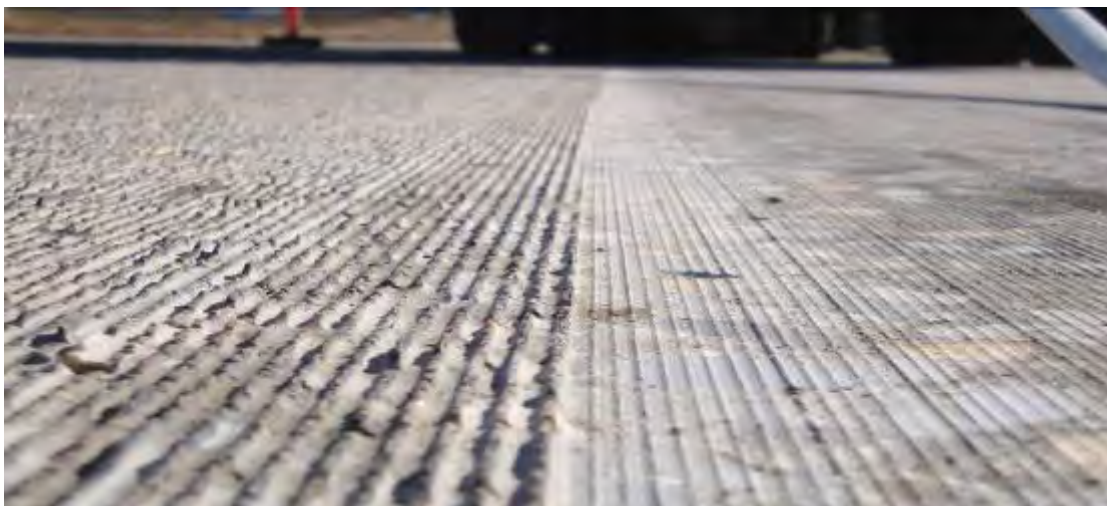
Figure 27. Conventional diamond grind on left with fine grind of NGCS on right before grooves were cut.
