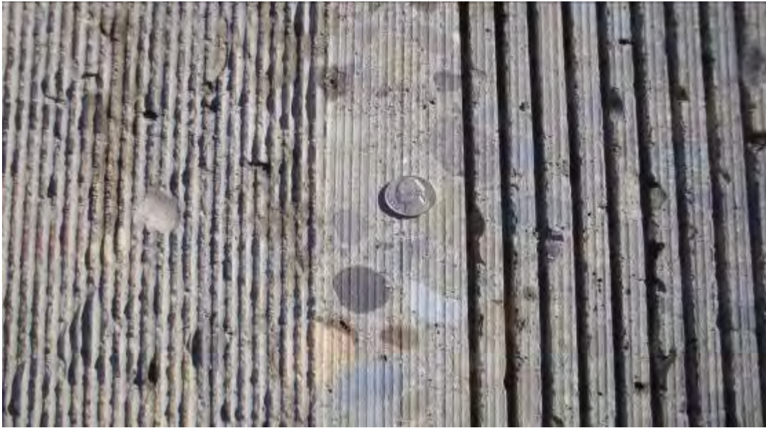
Figure 28. Conventional grind on left, fine grind in middle, and tall grind (complete NGCS) on right.
