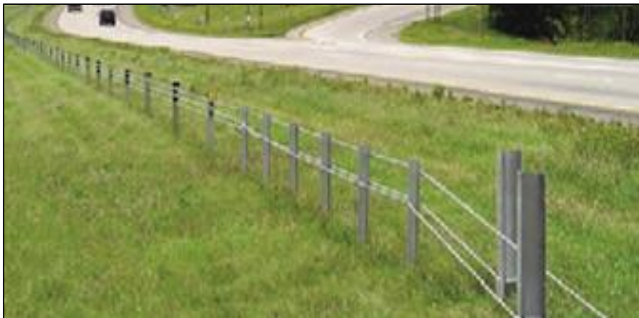
Figure 2.3 Trinity Cass TL-3 Cable Median Barrier System
