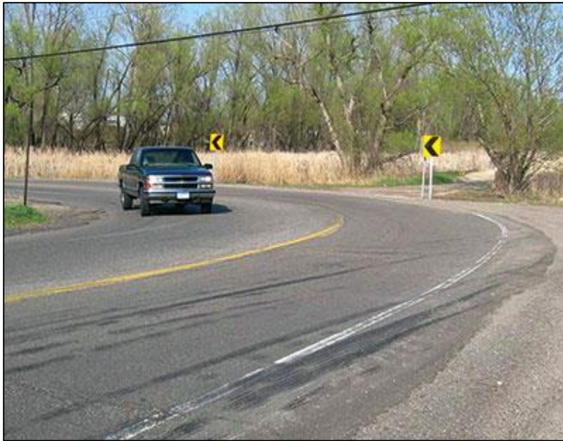
Figure 2.1 Shoulder Widening and Advanced Warning Signs on Horizontal Curves
