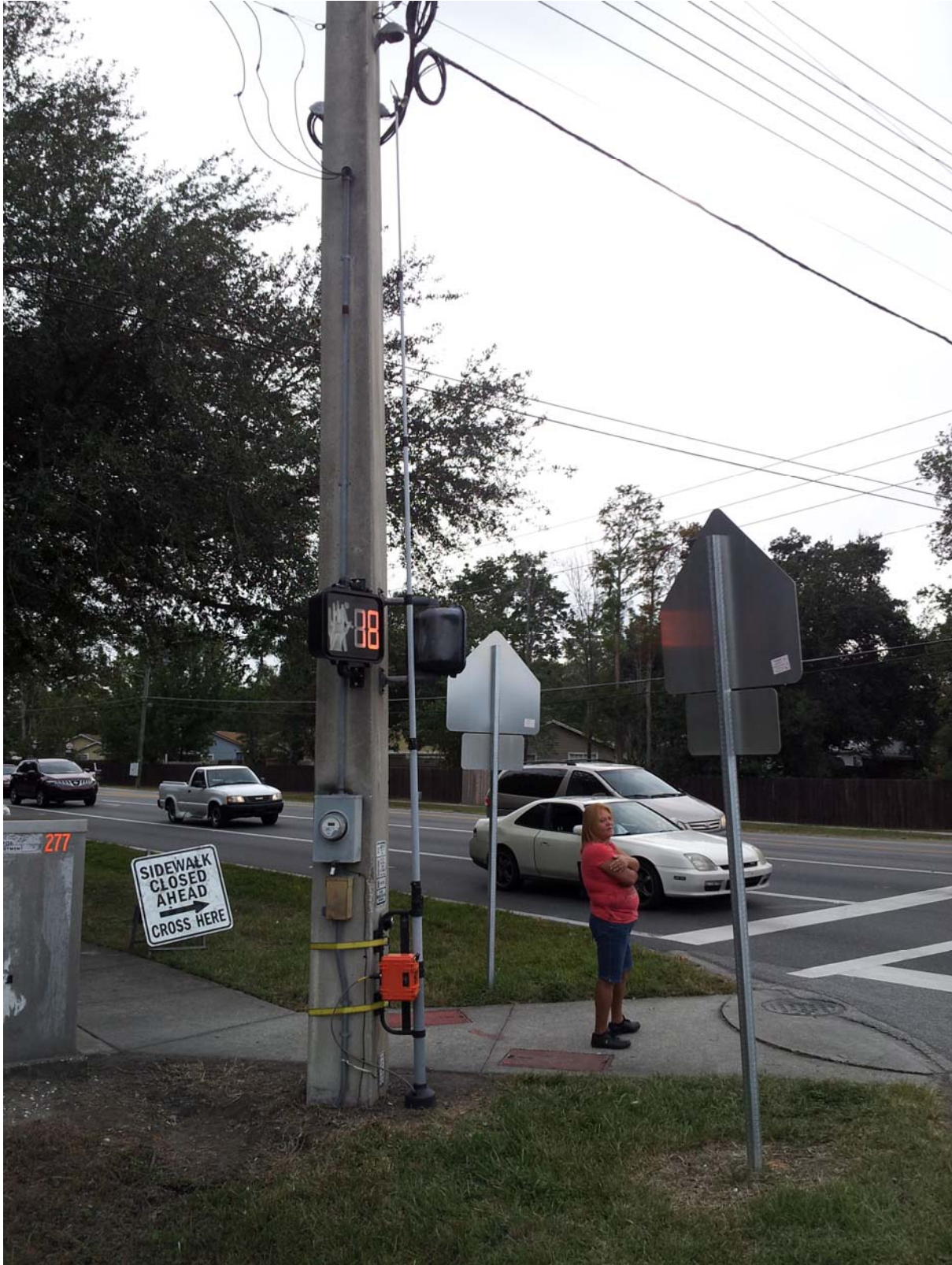
Scout VCU Unit attached to an electric pole with camera at 20 feet high @ Chickasaw Trail and Valencia College lane Intersection
