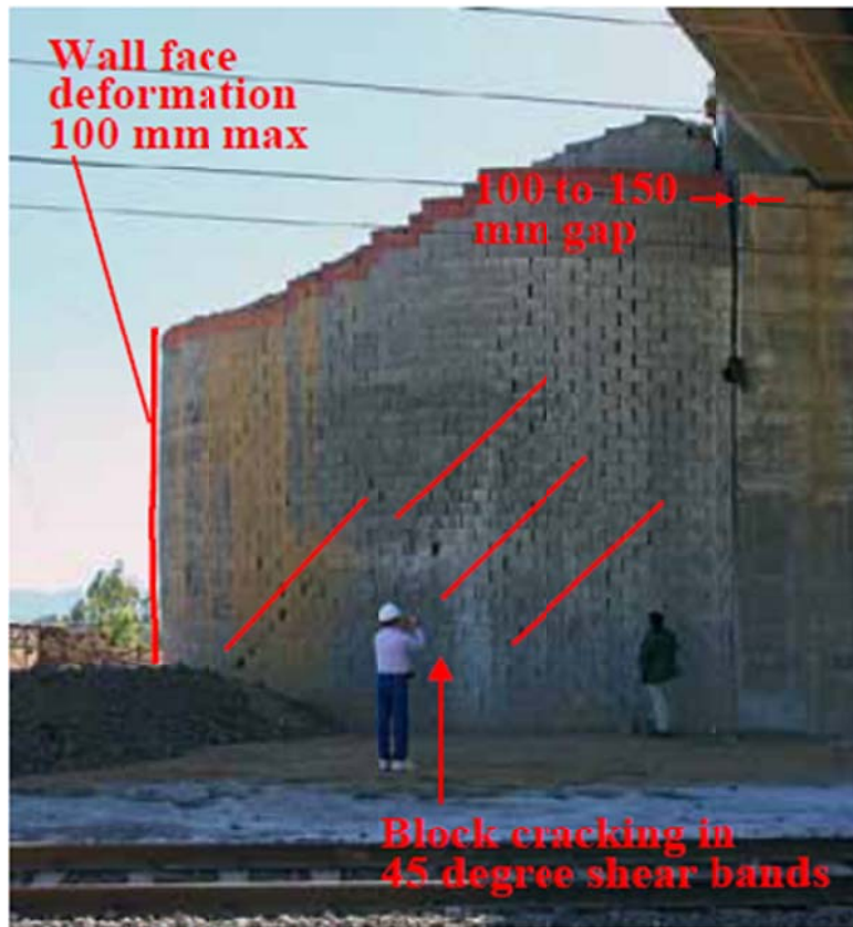
Figure 3-1: Wall cracked blocked pattern in 45 degree shear bands
