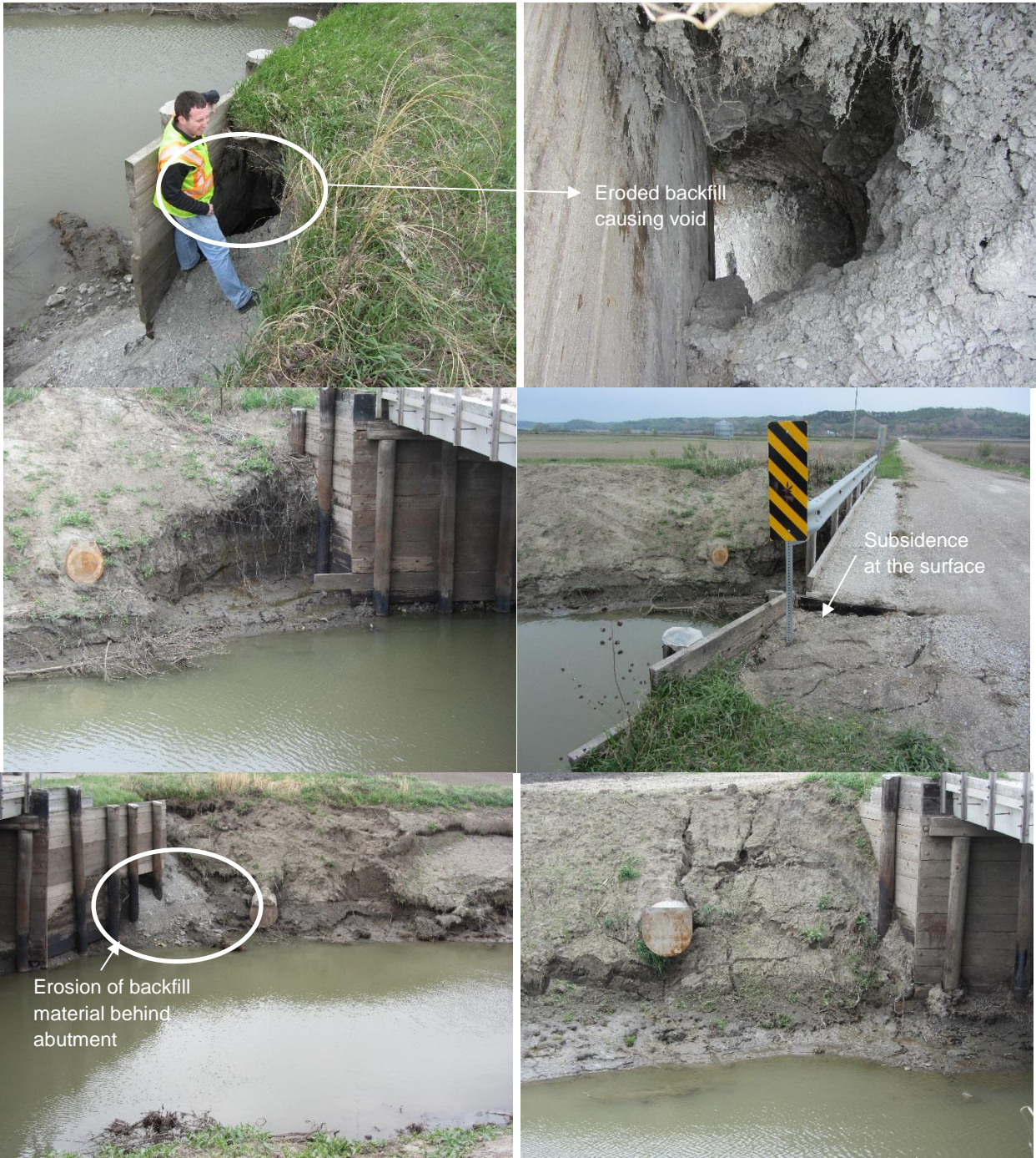
Figure 134. Bridge conditions on TS1 on 4/4/12 – Fremont County
