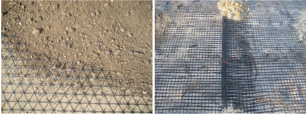
Figure D34. Triaxial (left) and biaxial (right) polymer geogrids placed on the subgrade
