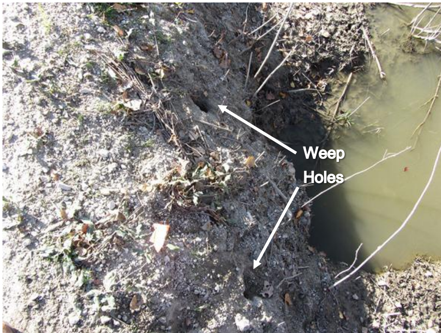
Figure 73. Weep holes near culvert on TS3 (Photo taken on 10/25/2011) – Pottawattamie County
