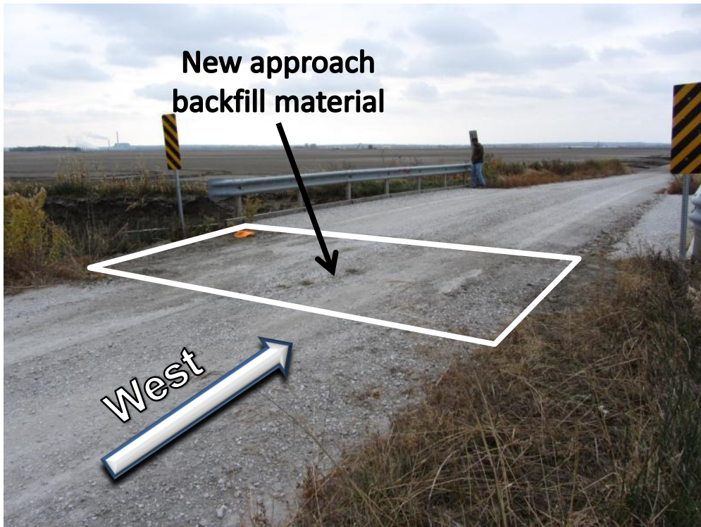
Figure 130. New bridge approach backfill material placed along the east approach on TS1 (Picture taken on 10/26/11) – Fremont County
