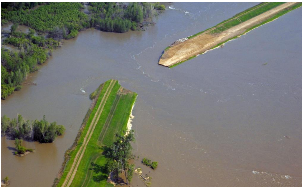
Figure 11. Aerial photo of the full breach at Federal levee 575 near Hamburg, Iowa, on June 14, 2011 (Image Courtesy of USACE http://www.flickr.com/photos/usacehq/5837117182/in/photostream/ )
