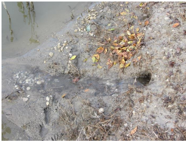
Figure 47. Weep holes detected under a gravel road – Meadowlark Loop Road, Pottawatomie County (Photos taken on 9/22/11)
