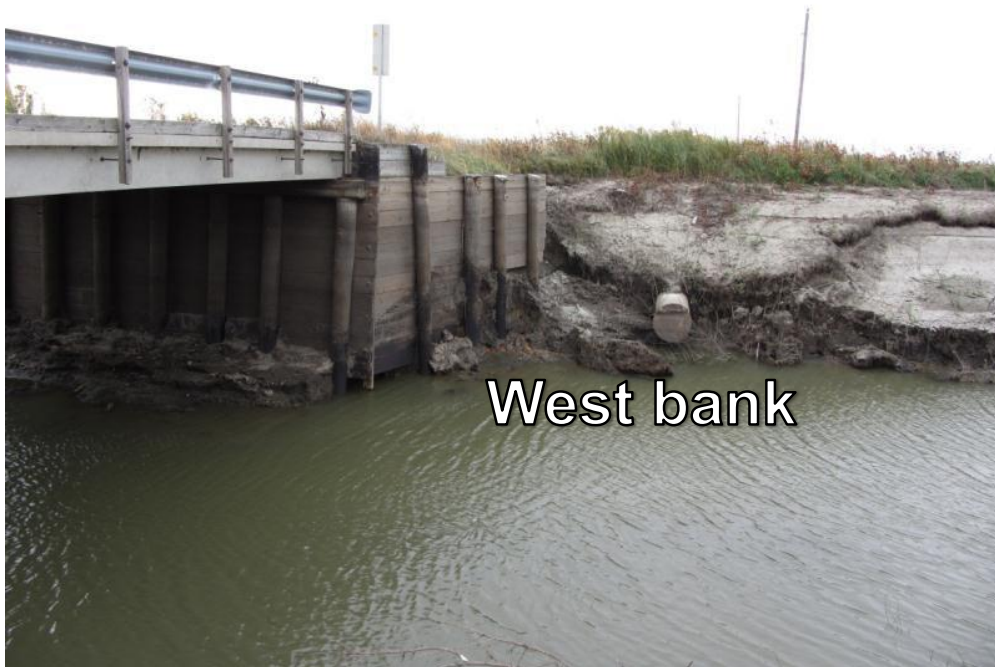
Figure 131. Erosion of embankment material along the west bank on TS1 (Picture taken on 10/26/11) – Fremont County
