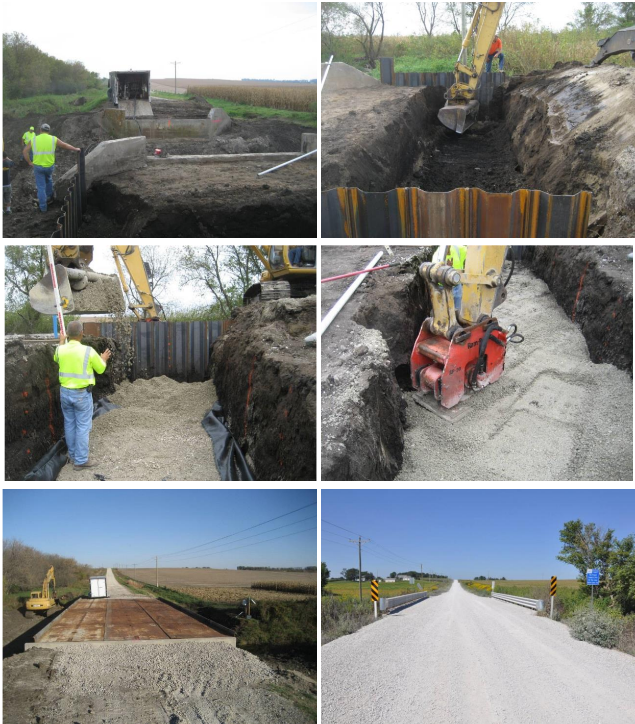
Figure D40. Pictures of a bridge site in Buchanan County (250 th Street) during construction of GRS fill in bridge abutments, placement of rail road flat cars for superstructure, and after final placing the final gravel surface in 2011 (Vennapusa et al. 2012)
