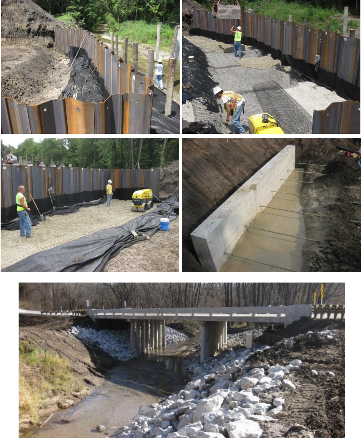
Figure D37. Pictures of a bridge site in Boone constructed with sheet pile abutments with geogrid-reinforced backfill material (Evans et al. 2012)
