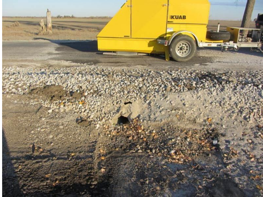
Figure 163. Surface patch repair over a culvert on TS4 – Fremont County (Picture taken 10/28/11)
