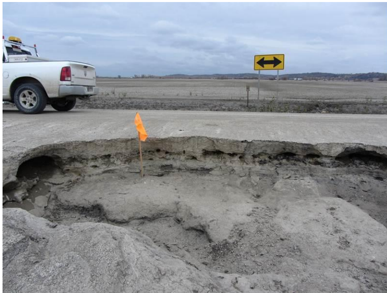
Figure 49. Erosion of shoulder and roadbed on a chip seal surfaced gravel road – Fremont County (Photo taken on 10/26/11)
