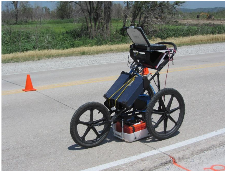
Figure 67. GPR scanning setup with 400 MHz antenna along the south side of the east bound lane on TS2 – Pottawattamie County
