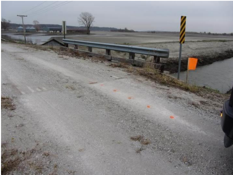
Figure 145. Bridge approach on TS2 (Picture taken 10/26/11)
