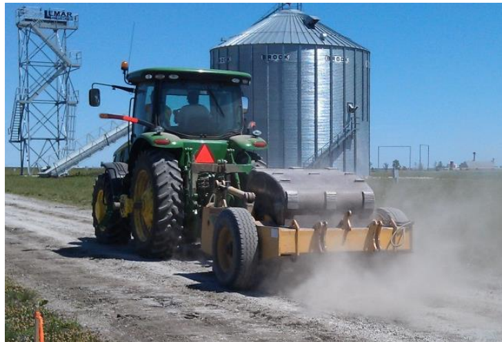
Figure D35. High energy impact roller (equipment by Impact Roller Technology, Plattsmouth, Nebraska)
