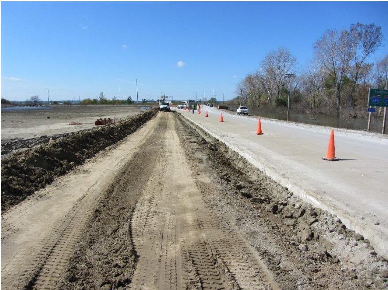
Figure 41. Eroded shoulder next to PCC pavement being reconstructed on 9/21/11 – Old Mormon Road (looking west towards I-680 and I-29 intersection), Pottawatamie County (Photos taken on 9/21/11)
