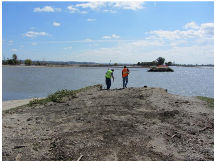
Figure 45. Full breach of about 150 m (500 ft) long unsurfaced access road – Pottawatamie County (Photo taken on 9/21/11)
