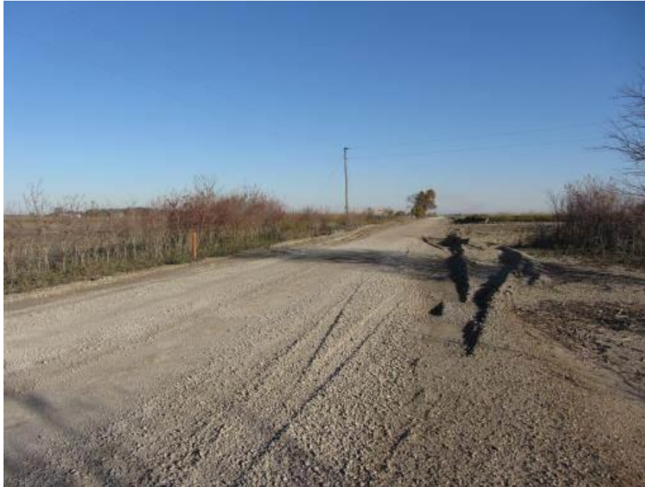
Figure 155. Newly placed gravel near a culvert at about 4700 m station on TS2 (Picture taken 10/27/11)
