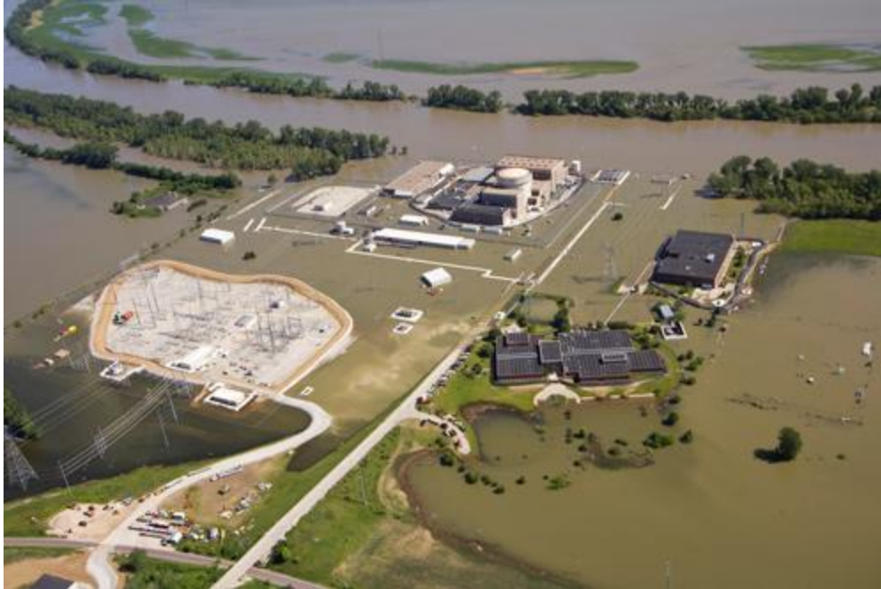
Figure 12. Aerial photo of the flooding near the Fort Calhoun nuclear power plant near Blair, Nebraska on June 17, 2011 (Image Courtesy of Omaha Public Power District)
