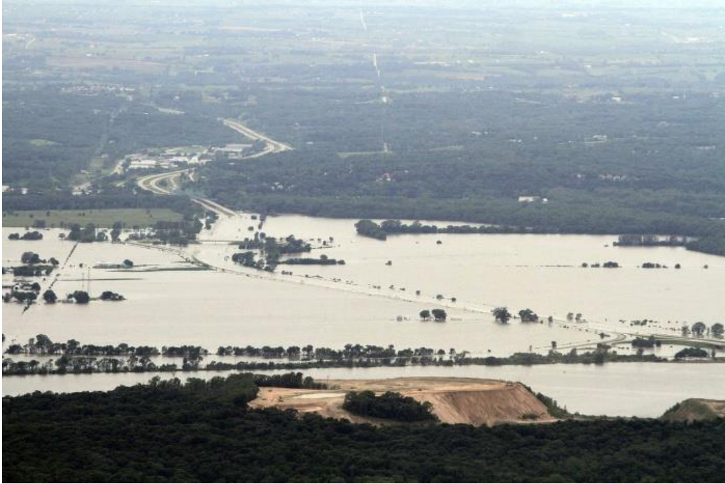
Figure 10. Aerial photo of the flooding on I-29 between Council Bluffs and Hamburg, Iowa on June 16, 2011 (Image Courtesy of Rodney White, The Register)
