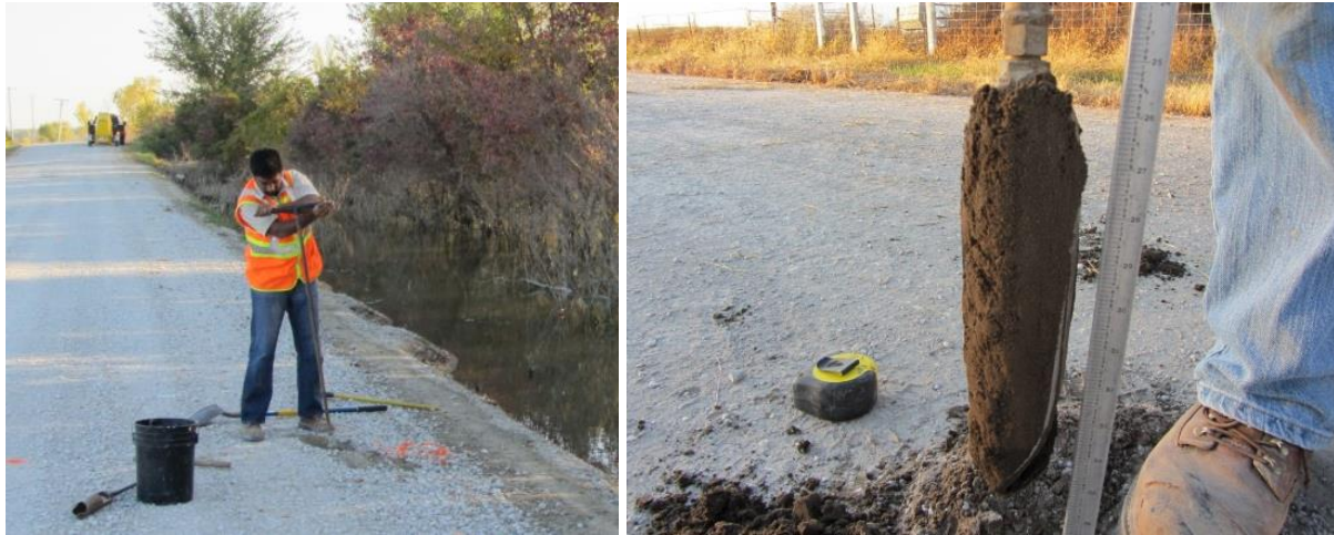
Figure 24. Extracting soil samples using a hand auger equipped with a Dutch auger head
