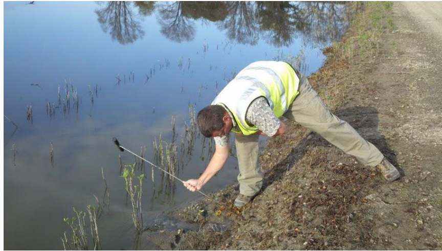
Figure D8. Hand push T-bar to inspect weep hole
