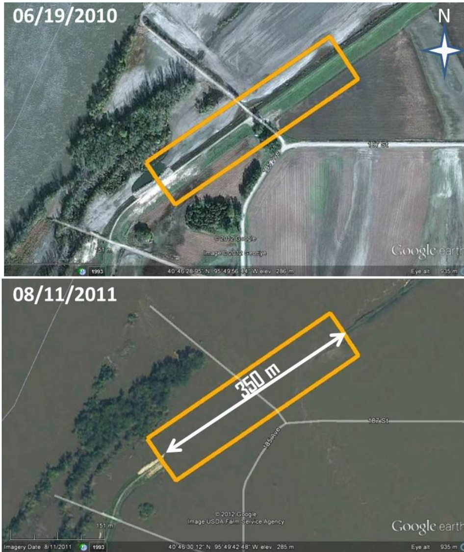
Figure 35. Levee breach in north part of Fremont County (images updated on 6/9/10 and 8/11/11)
