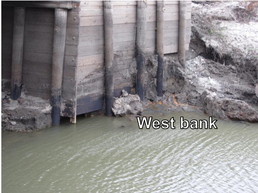
Figure 132. Erosion of embankment material along the west bank near abutment wing walls on TS1 (Picture taken on 10/26/11) – Fremont County
