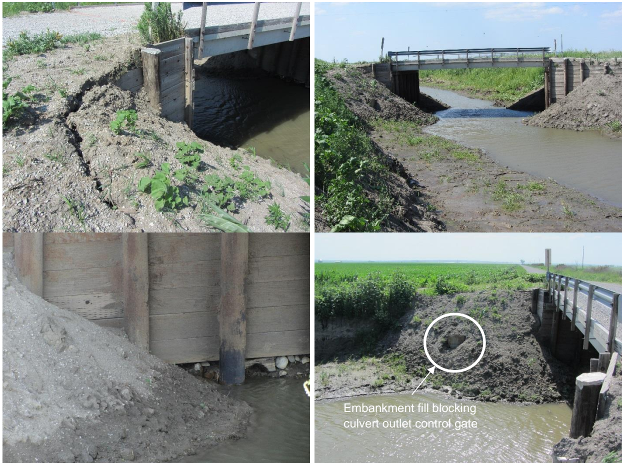
Figure 135. Bridge conditions on TS1 on 6/9/12 – Fremont County
