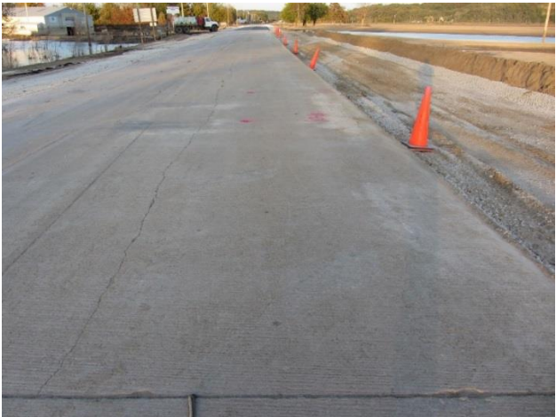
Figure 64. Longitudinal cracks on PCC pavement with undermined base material on TS2 (Photo taken on 9/21/11) – Pottawattamie County
