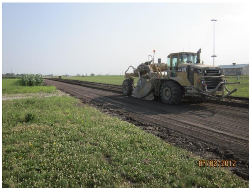
Figure D32. Blending granular material with subgrade using a soil pulverizer
