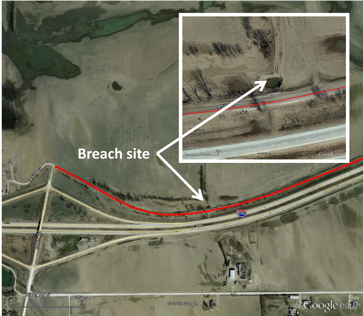
Figure 97. Aerial imagery of the breach site located next to TS5 145th St. (Google image from 3/7/12) – Pottawattamie County
