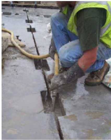
Figure 2–7. Pumping W.R. Meadows Sealign CG-86 non-shrink grout (Source: Oliva et al. 2007)
