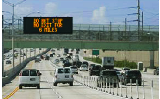
THE HOV lanes (center) on this stretch of I-95 could be used to manage traffic after an incident on the general purpose lanes (right).
