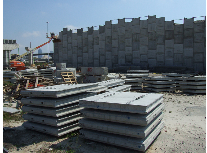
MSE wall being constructed from concrete panels for an overpass in Jacksonville.
