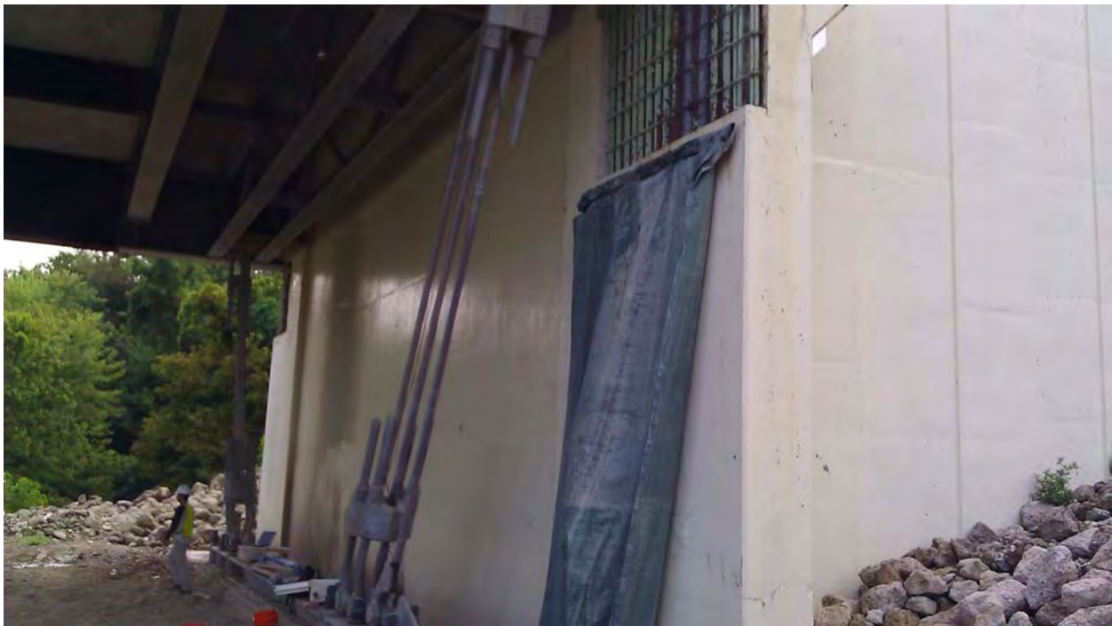
Figure 6.21: Pulldown Rehab at Kentucky Abutment, USG, 2011
