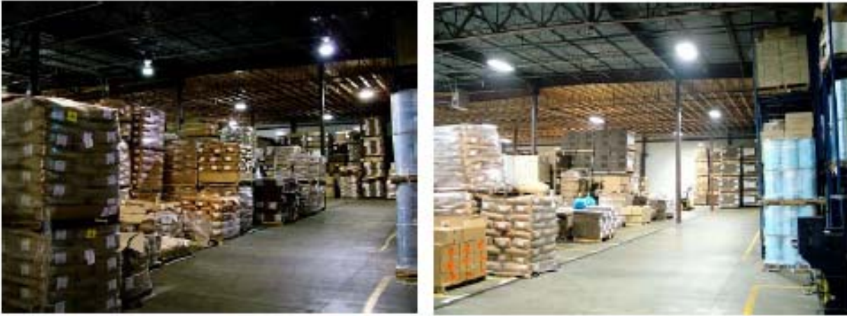
Figure 4.25. Before and after pictures of a Trident Seafood facility where MH lamps were replaced with HIF lamps (Seattle Government- Energy Smart Services).
