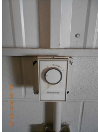
Figure 4.13. Dial control for setting radiant heaters' temperature.
