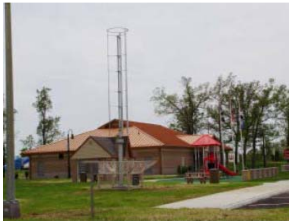
Figure 3.10. Vertical-axis turbine. Source: http://www.windspireenergy.com/case-studies/missouri-department-of-transportation/attachment/mdot_2/
