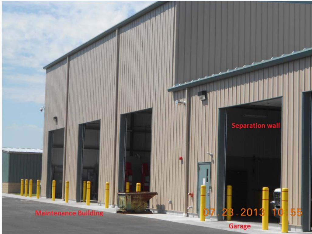
Figure 5.2. Maintenance area and garage area are thermally separated by a wall in the New Lucas County Garage.
