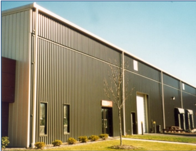
Figure 6.6. Brown collector on industrial building, Connecticut, USA. Photo credit Conservall Engineering.
