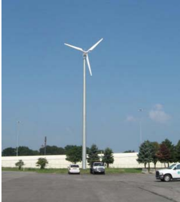
Figure 3.9. Horizontal axis turbine at ODOT Northwood outpost facility
