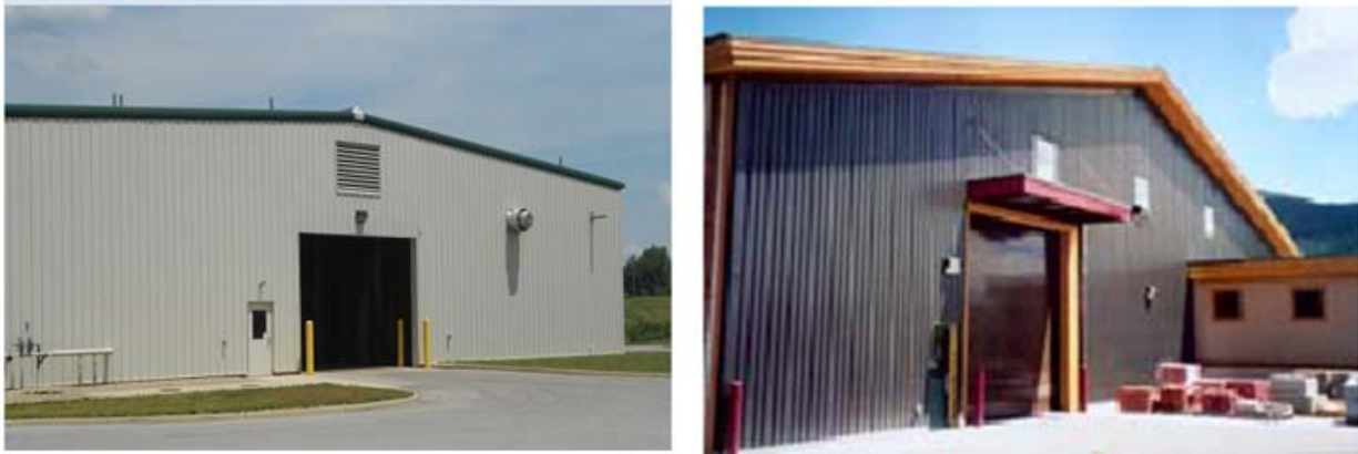
Figure 4.29. The southern facing wall of the Pike County Garage and a solar air heating system installed on a similar wall.
