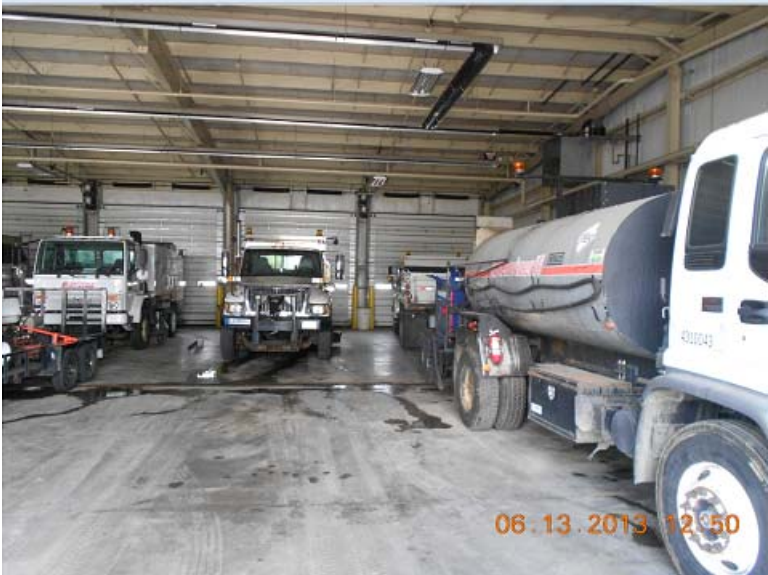
Figure 4.26. Fifth avenue outpost garage use HID fluorescent fixtures in the garage area.
