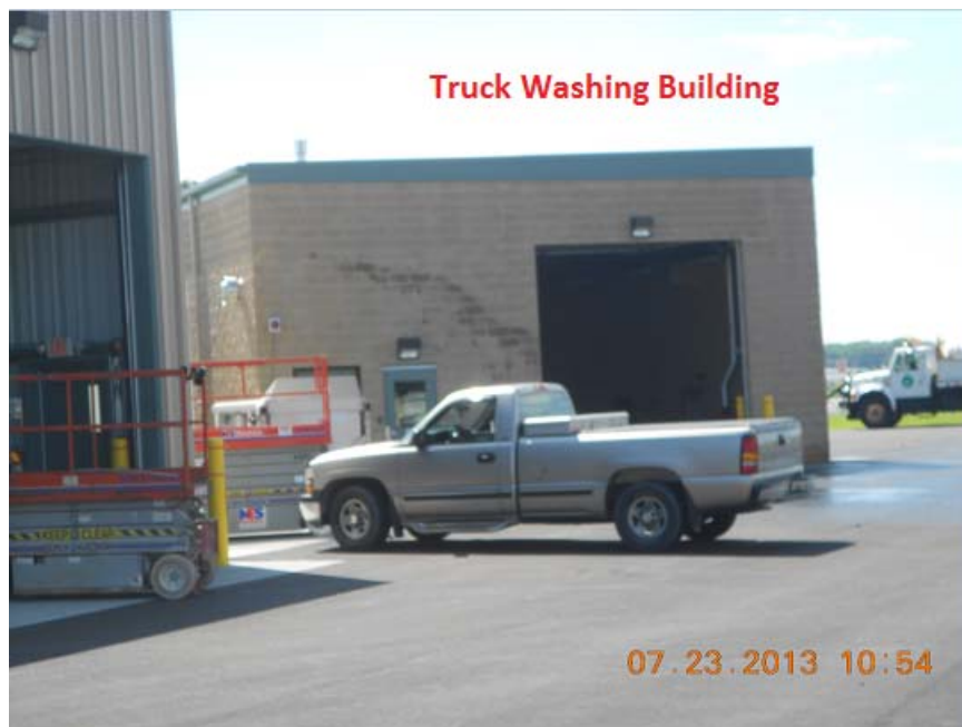
Figure 5.3. A separate truck washing building is used in the New Lucas County Garage
