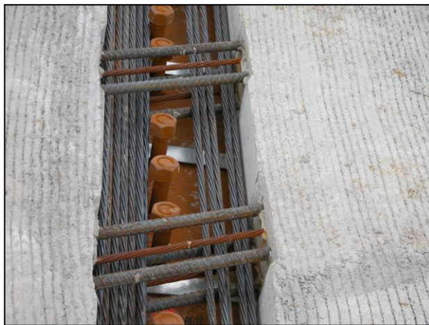
Figure 1.2: Threading post-tensioning strands (left) and conflicts between deck reinforcement and shear connectors (right)
