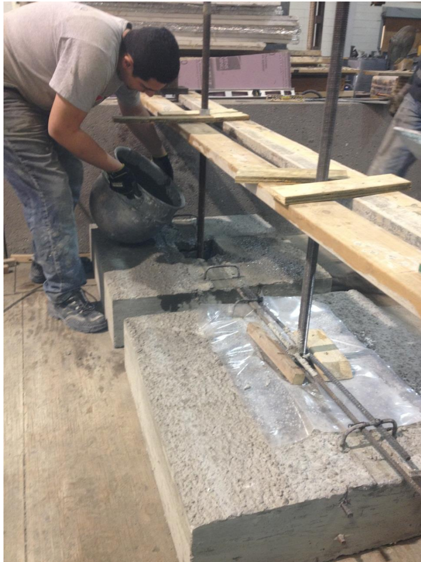
Figure 5.22: Filling the pockets using commercial grouts
