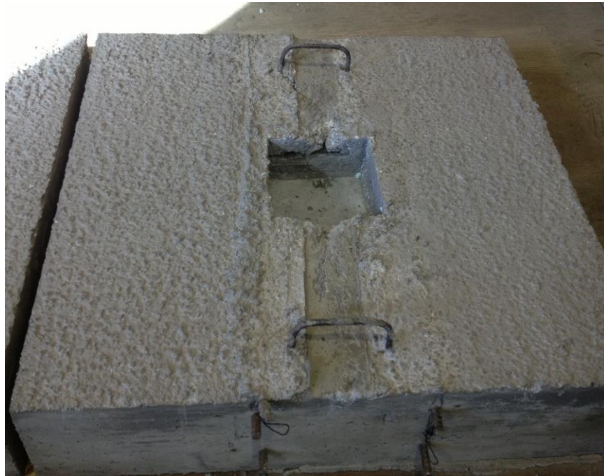
Figure 5.21: Foam blockout used to form the pocket in deck specimens
