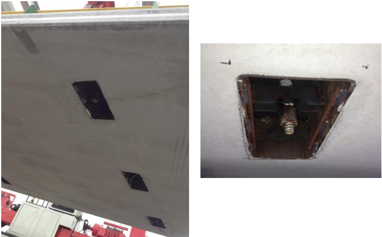
Figure 6.8: Photos of the soffit of the demonstration panel during lifting
