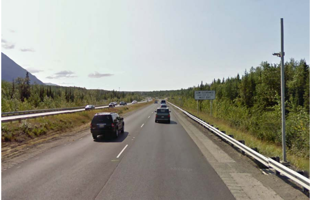
Figure 2 Southbound Overheight Detector (Source: Street View Google Maps ©2011 Google)
