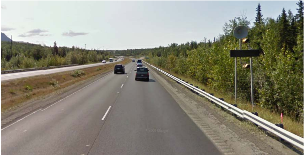
Figure 3. Southbound Freeway Mainline Blank Out Sign and Alarm Speaker (Source: Google Maps ©2011 Google)
