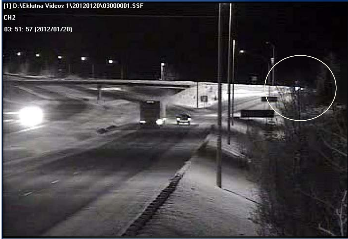
Figure 12 The VMS during flashing (located in center of the circle area)
