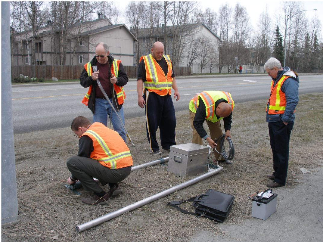
Figure 2. Photo. Pole-mount System Installation
