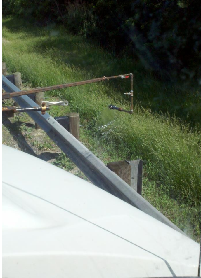
Figure 4.14: Epoke Spraying Guardrail with Herbicide.
