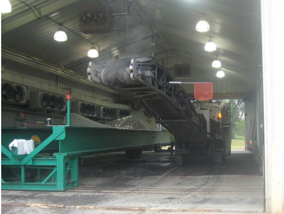
Figure 8.4: Milling of Pavement Sections.
