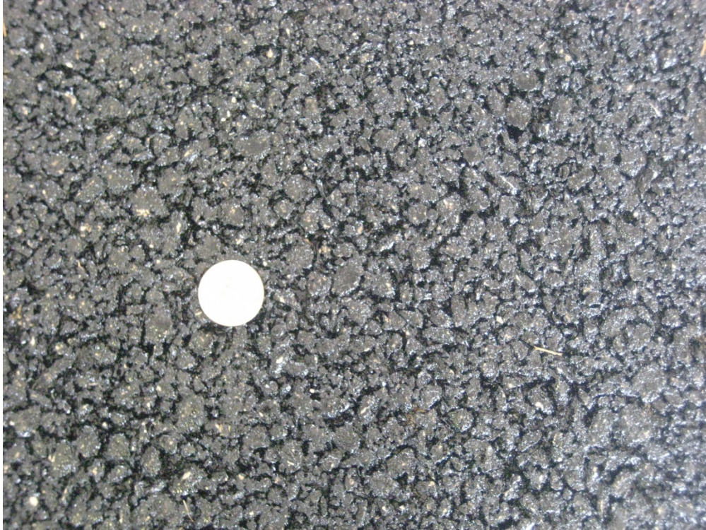
Figure 8.10: Picture of the Compacted Surface Course.
