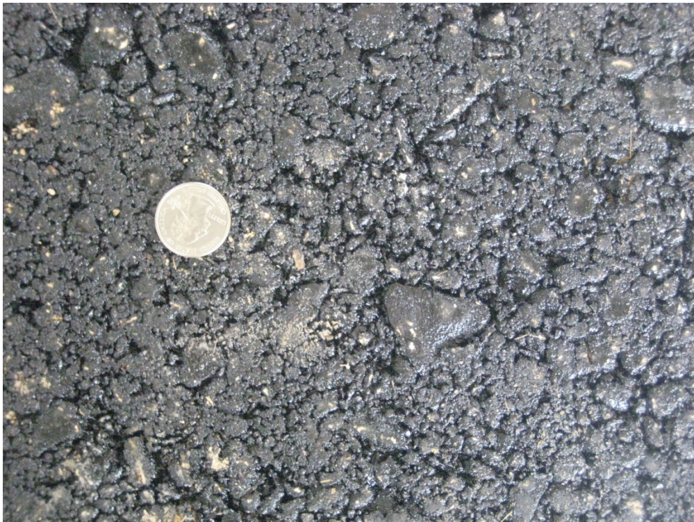
Figure 8.11: Picture of the Compacted Intermediate Course.
