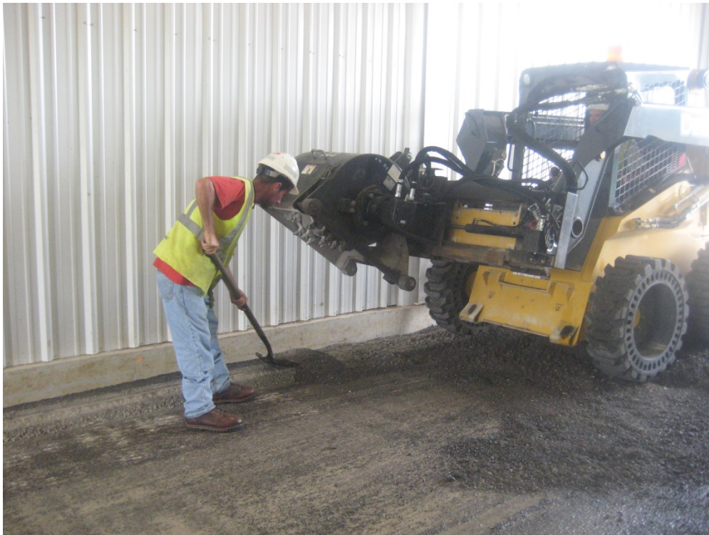
Figure 8.5: Cold Milling Machine Near Edges.
