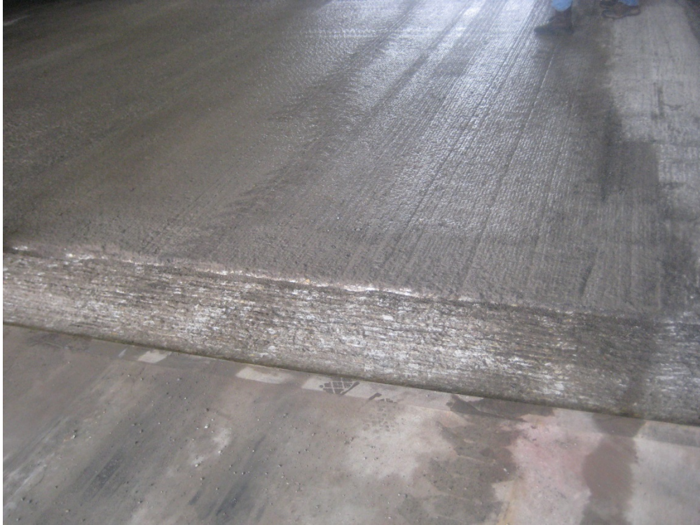
Figure 8.6: Milled Pavement Surface.
