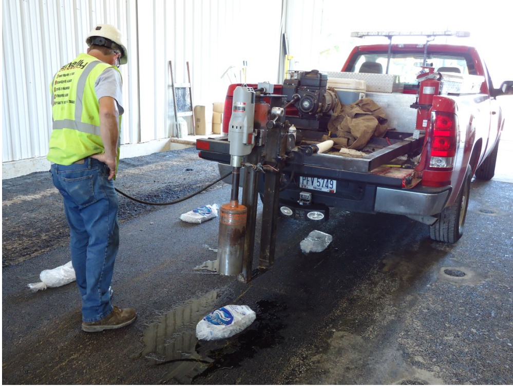
Figure 8.12: Coring of Field Specimens.
