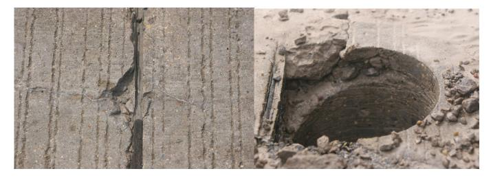
(a) (b) Figure 3.6 (a) WB, I-94, transverse joint spalling deterioration at intercept of longitudinal crack from vibrator trails, and (b) deterioration initiation just below the tined surface from mortar erosion.
