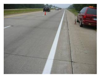
Figure 3.3 WB I-94, Lawrence, MI, showing end of section without joint distress and the beginning of the section with distress.
