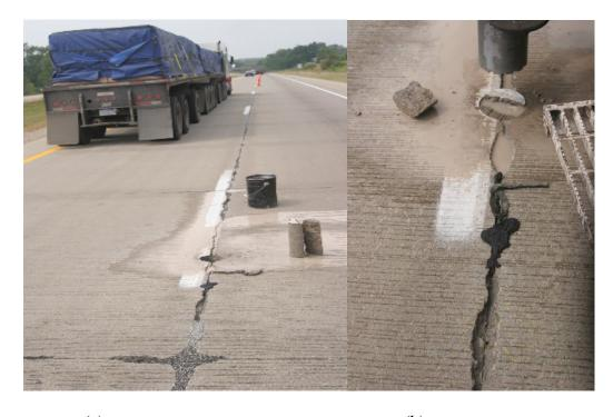
(a) (b) Figure 3.7 WB I-94, Lawrence, MI, with longitudinal joint deterioration (a), and (b) poorly draining joint.
