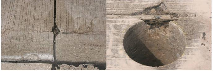
Figure 3.5 Close-up of joint deteriorated concrete (WB, I-94, Lawrence, MI).
