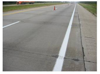
Figure 3.2 Transverse joint staining and spalling near outside shoulder (WB, I-94, Lawrence, MI).
