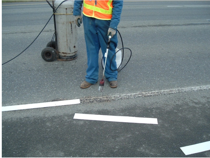
Figure 34. Photo. Applying preformed thermoplastic.
