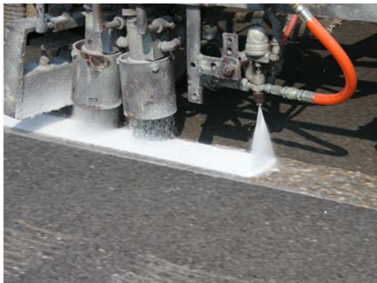
Figure 103. Photo. Close-up of pavement marking installation.
