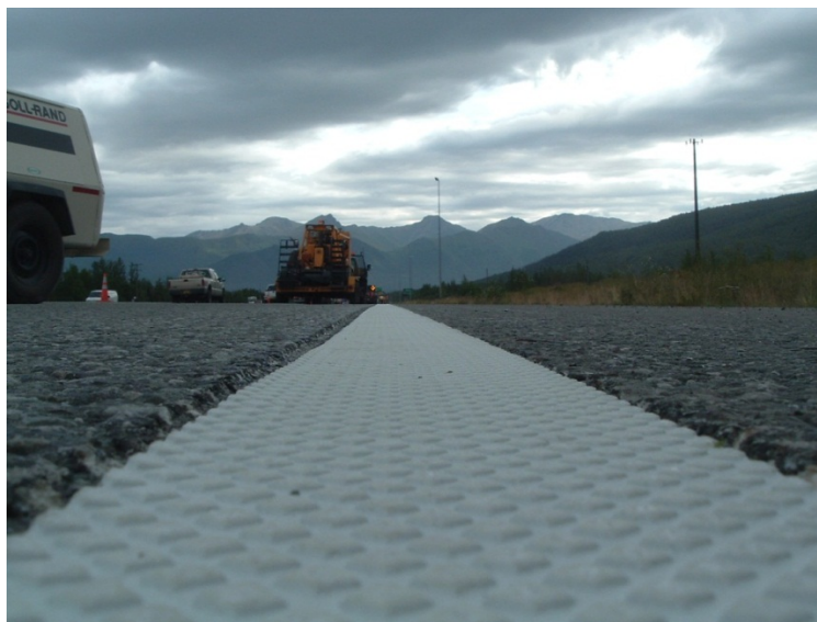
Figure 36. Photo. Marking tape in recessed pavement groove.
