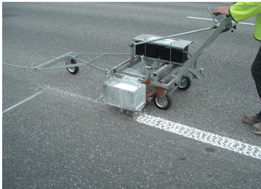
Figure 35. Photo. Applying structured MMA.
