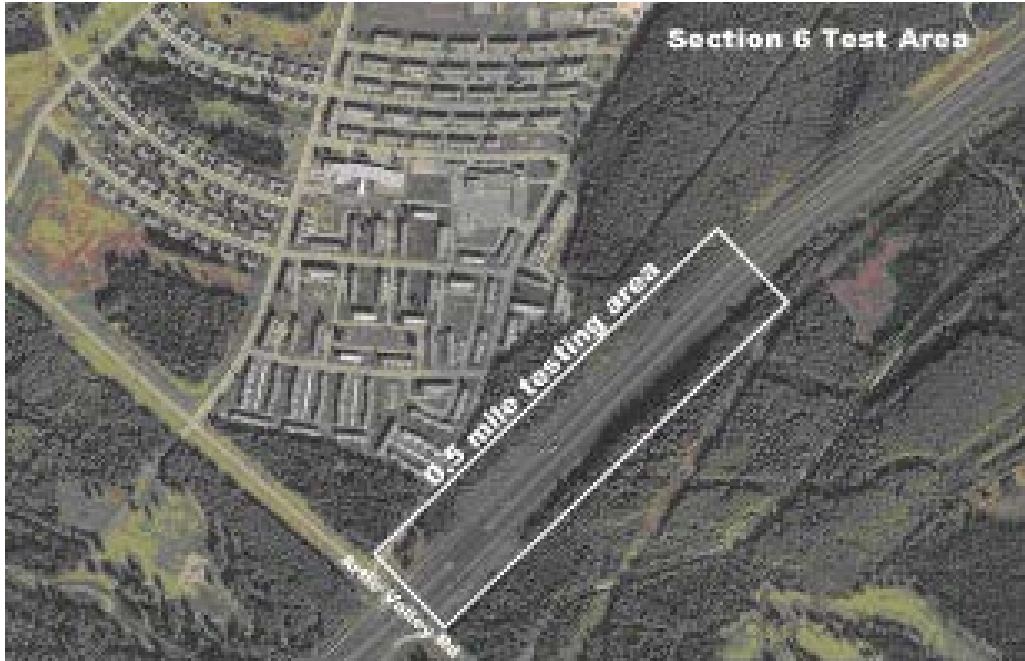
Figure 56. Photo. Test section 6 (Anchorage, AK).
