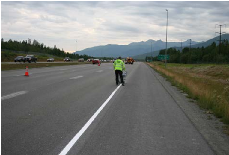
Figure 100. Photo. Pavement marking installed in Alaska in 2006.
