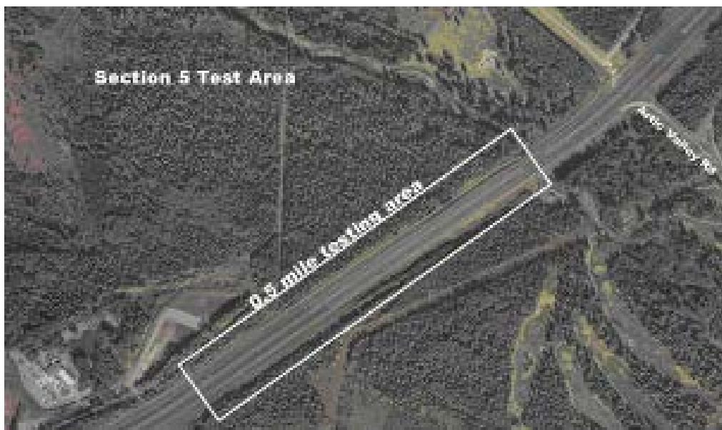
Figure 55. Photo. Test section 5 (Anchorage, AK).
