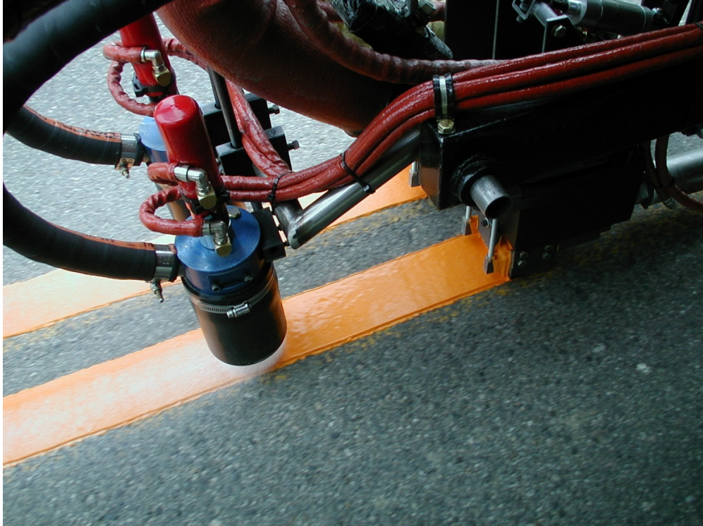
Figure 37. Photo. Glass beads applied with bead gun on thermoplastic.
