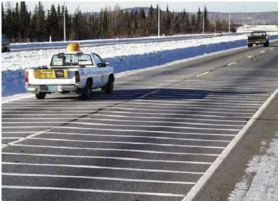
Figure 2. Photo. Transverse test deck in Alaska.
