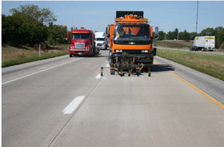
Figure 102. Photo. Pavement marking installation.
