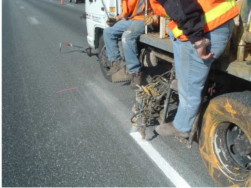
Figure 33. Photo. Applying paint with a truck sprayer.
