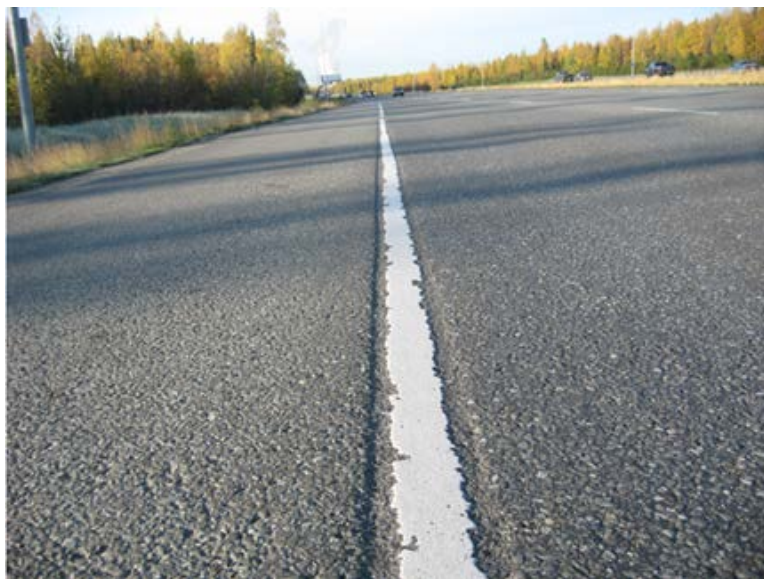
Figure 101. Photo. Pavement marking after 2 years in Alaska in 2008.
