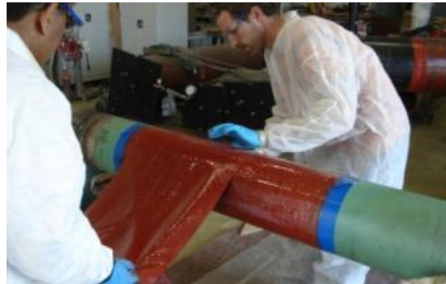
*Figure 30 - Application of the carbon wrap on the 8-inch pipe*
