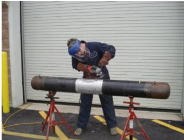
*Figure 29 - Surface preparation for the composite repair application*
