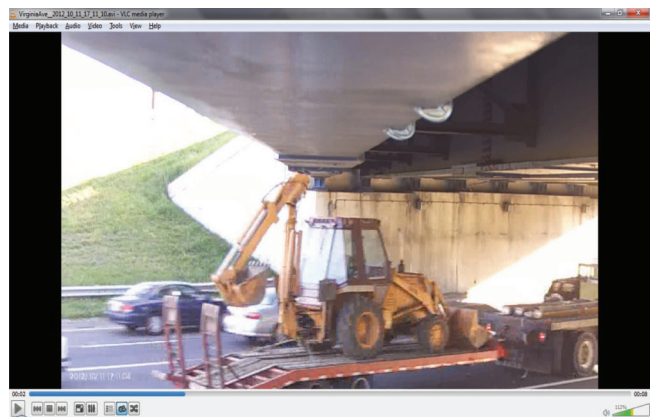
Figure 5.3 Image taken from video of a backhoe tractor impacting the Virginia Avenue Bridge in Indianapolis, Indiana.
