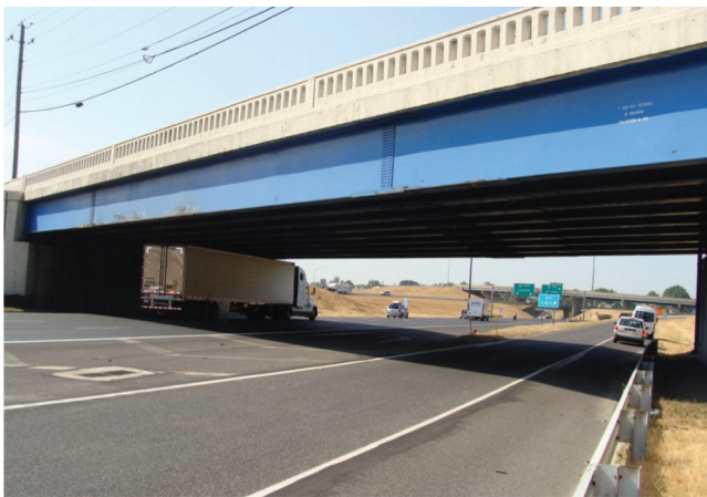
Figure 1.1 Virginia Avenue Bridge over I-65 SB in Indianapolis, Indiana (southern perspective).
