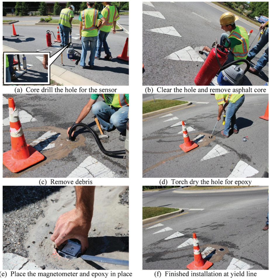
Figure 3.7 Installation of wireless magnetometer for entering vehicle.
