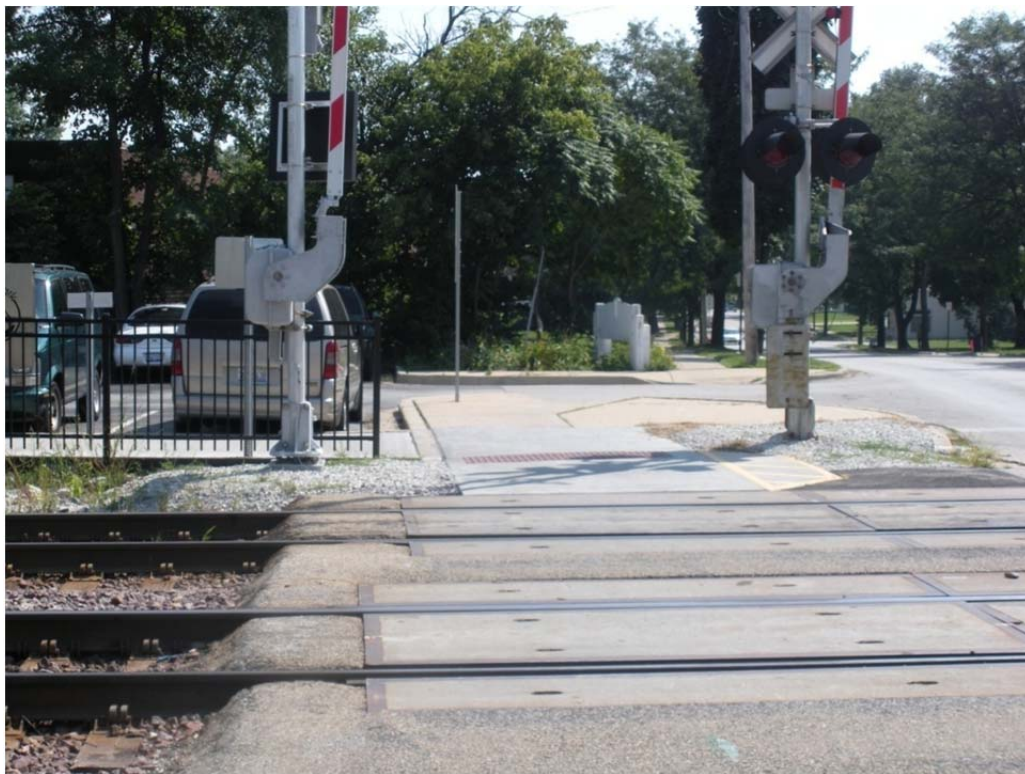
Figure 18. Crossing 174937L – A view from the ground.
