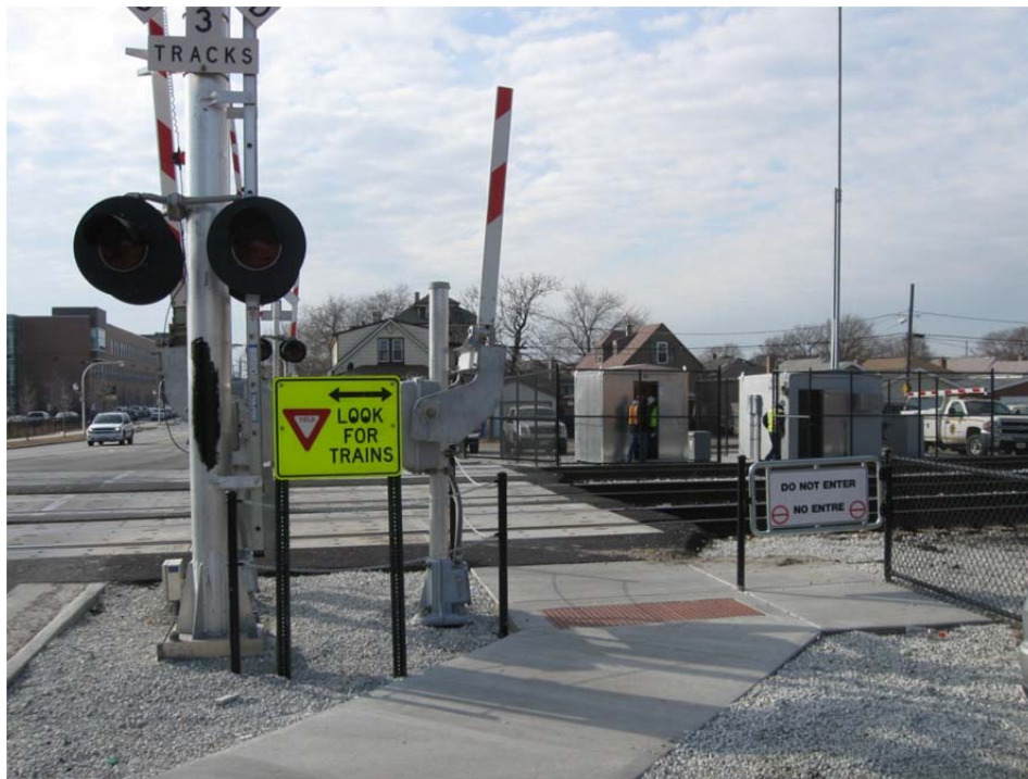
Figure 12. Crossing 843811C – A view from the ground (courtesy of ICC).
