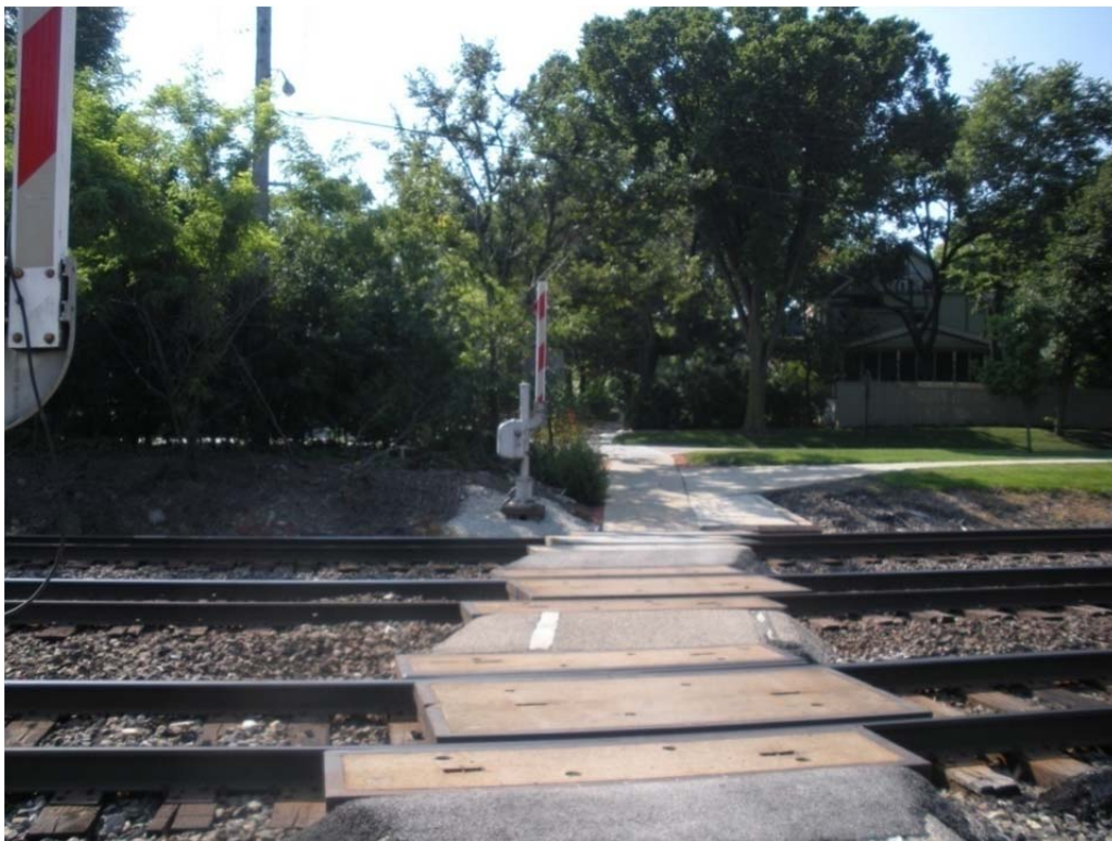
Figure 16. Crossing 079521M – A view from the ground.
