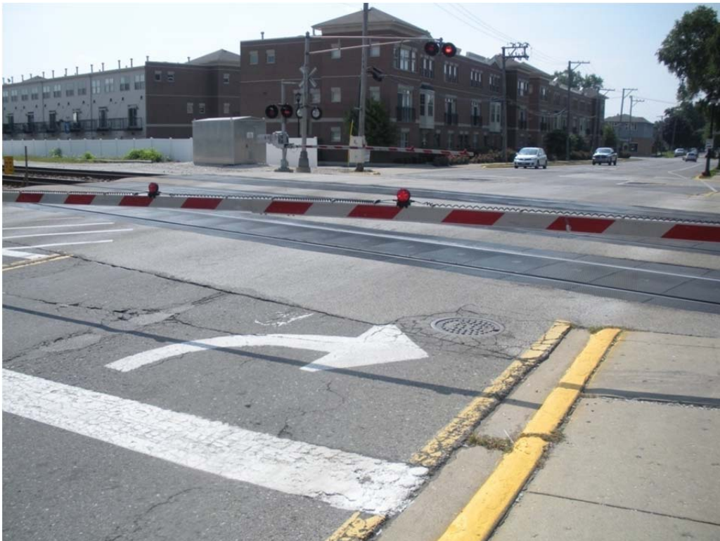
Figure 20. Crossing 372128W – A view from the ground.
