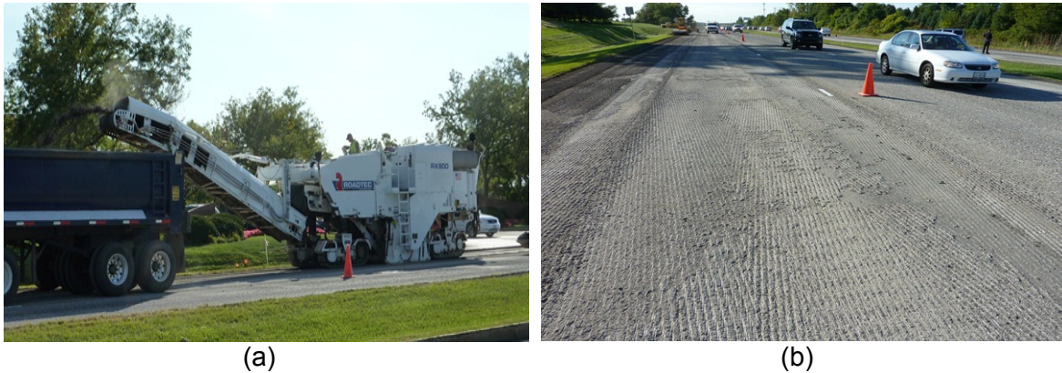
Figure 3. (a) Milling of old pavements, and (b) milled surface.
