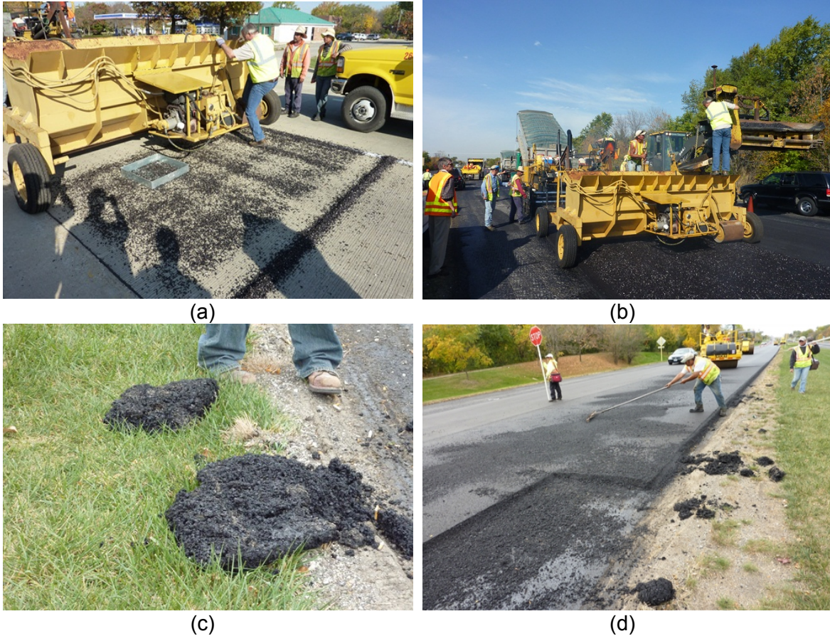
Figure 6. (a) Chip spreader, (b) feeding sprinkle chips from shoulder, (c) lump of slag/fiber mixtures, and (d) material supplements on the uneven surface.
