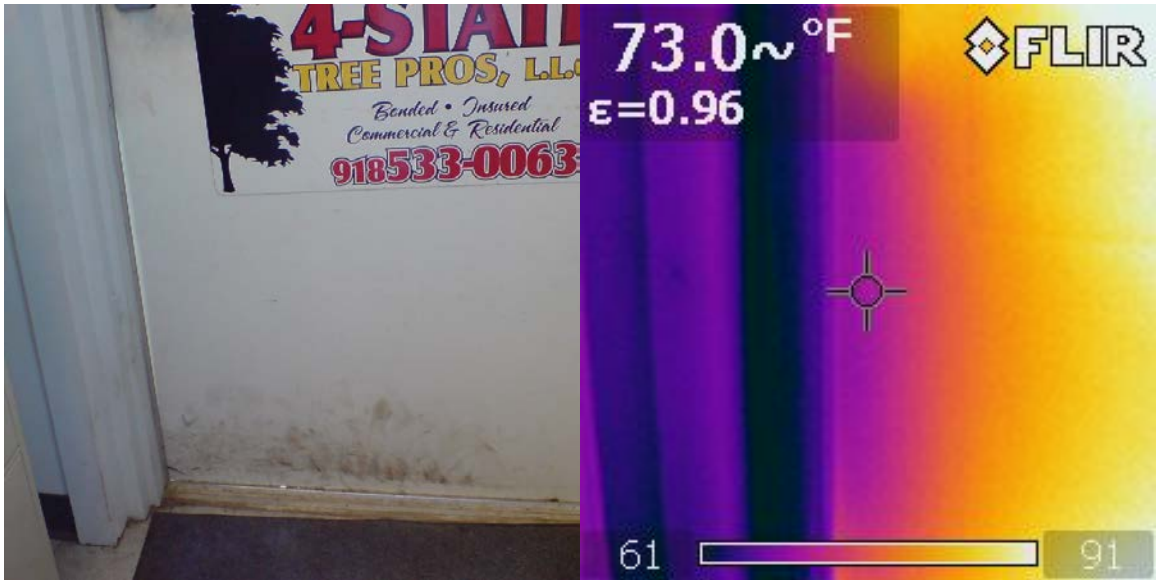
FIGURE 4.50 Infiltration Detection—Exterior Door
