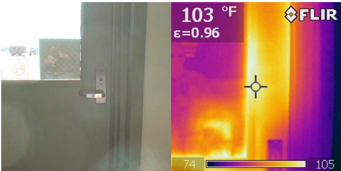
FIGURE 4.40 Infiltration Detection—Exterior Door
