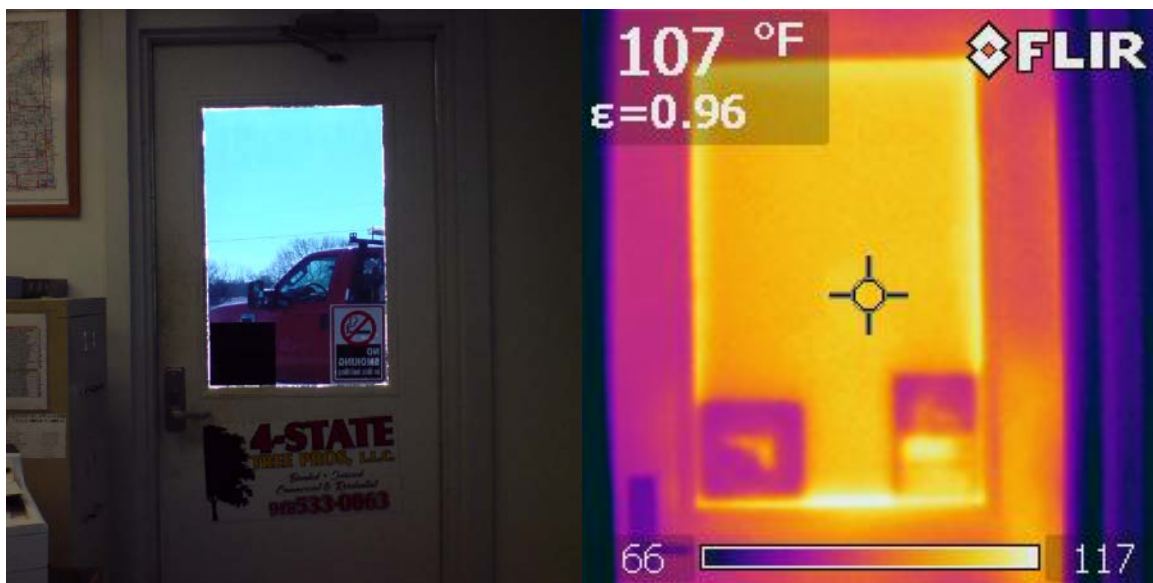
FIGURE 4.49 Infiltration Detection—Exterior Door
