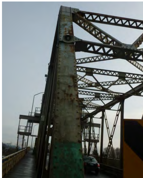
Figure 7. Southeast-bound US 101 Bridge
