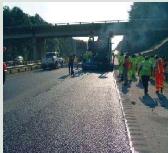
Figure 2 Workers laying down OGFC test sections
