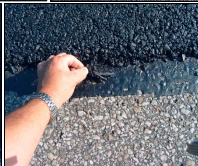
Figure 2 Construction of OGFC
