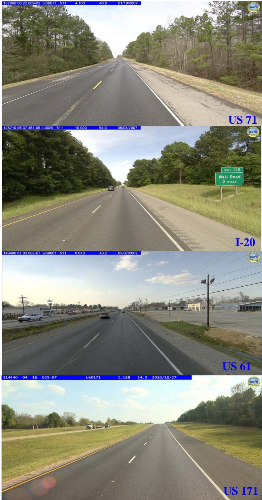
Figure 3 LADOTD OGFC test sections
