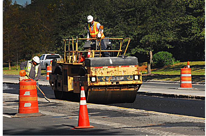
Vibratory compactors and pile drivers produce intense vibrations that can damage susceptible structures or sensitive equipment.
