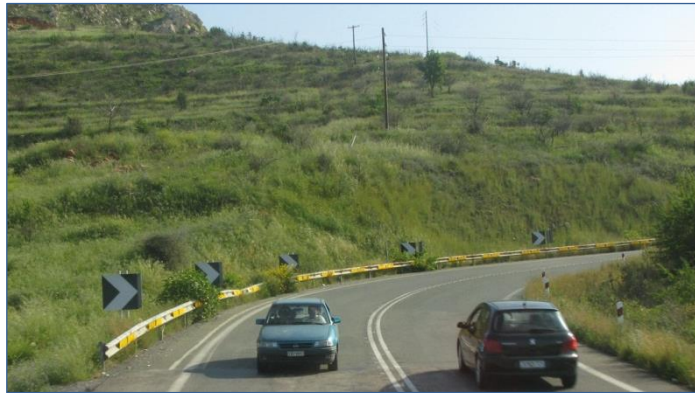
Figure 3. Panels of retroreflective sheeting to delineate curves
