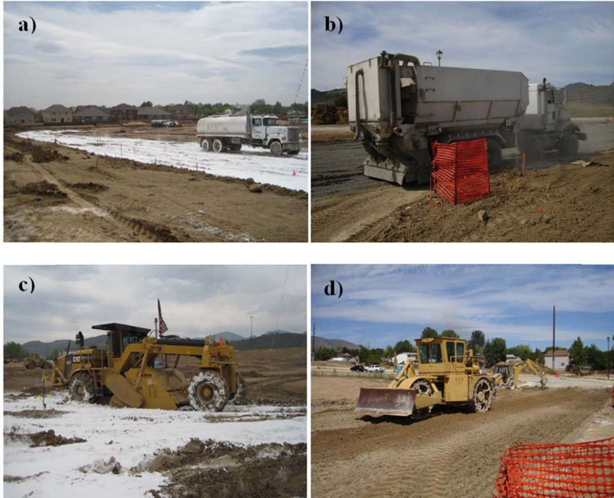
Figure 3.5: (a) Application of quicklime slurry, (b) application of cement, (c) soil/stabilizer mixing, and (d) final compaction.
