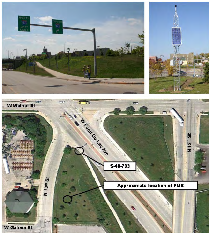
Figure 2.2 Location of Milwaukee sign support structure S-40-703 and the field monitoring station used to collect site/sign-specific wind data and corresponding bending strain response.
