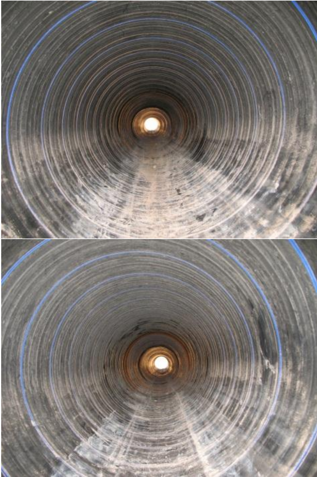
Figure 6. DuroMaxx pipe photos at initial visit; north pipe (top) and south pipe (bottom).
