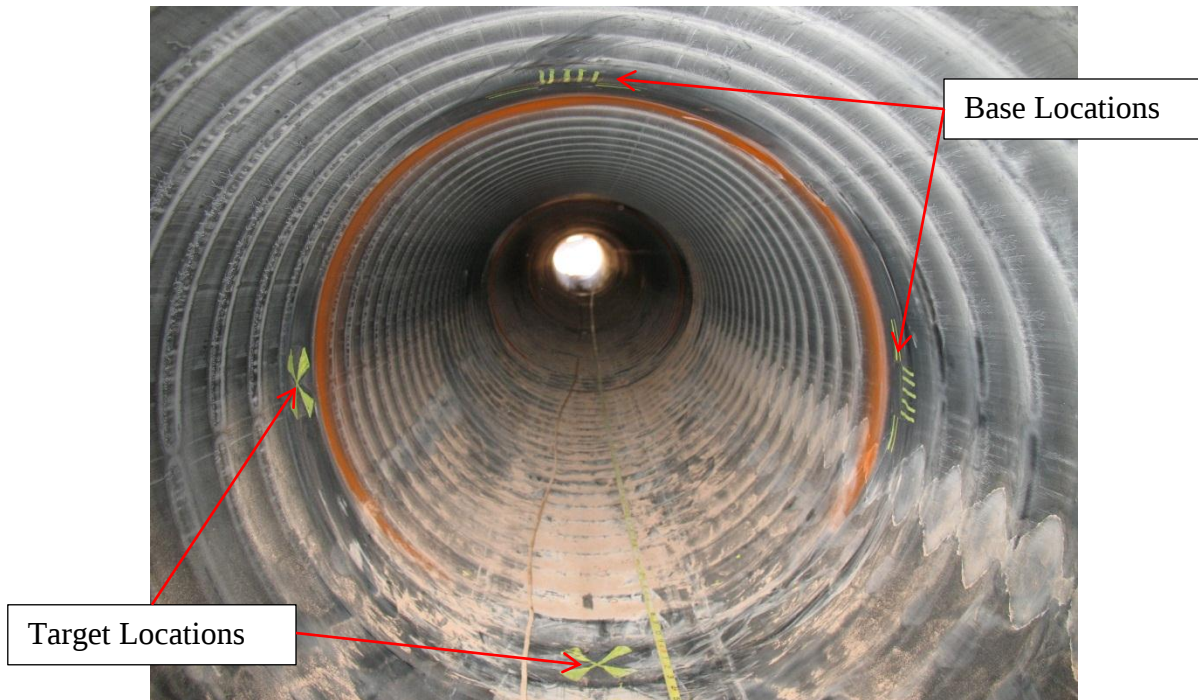
Figure 4. Base and target marking at a measurement station.
