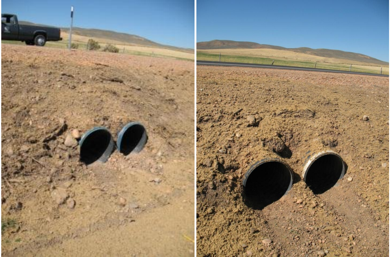
Figure 1. Photographs of the DuroMaxx (left) and ADS (right) pipe installations.
