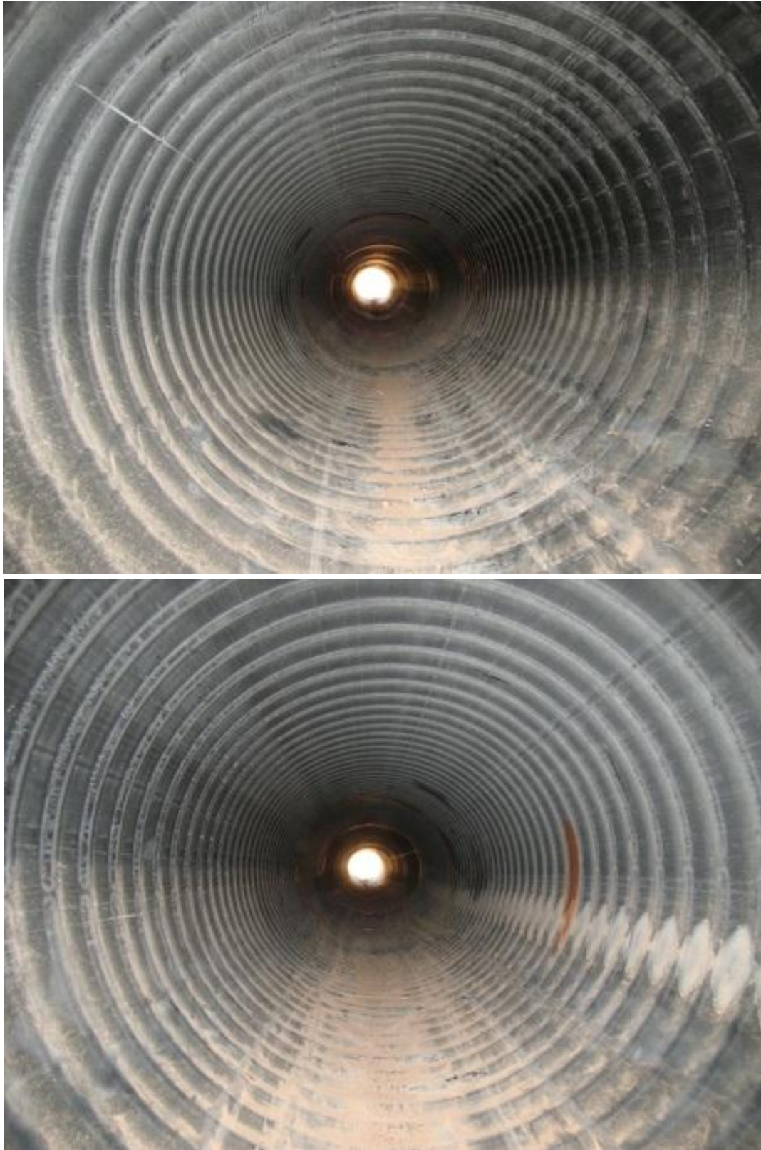
Figure 7. ADS pipe photos at initial visit; north pipe (top) and south pipe (bottom).
