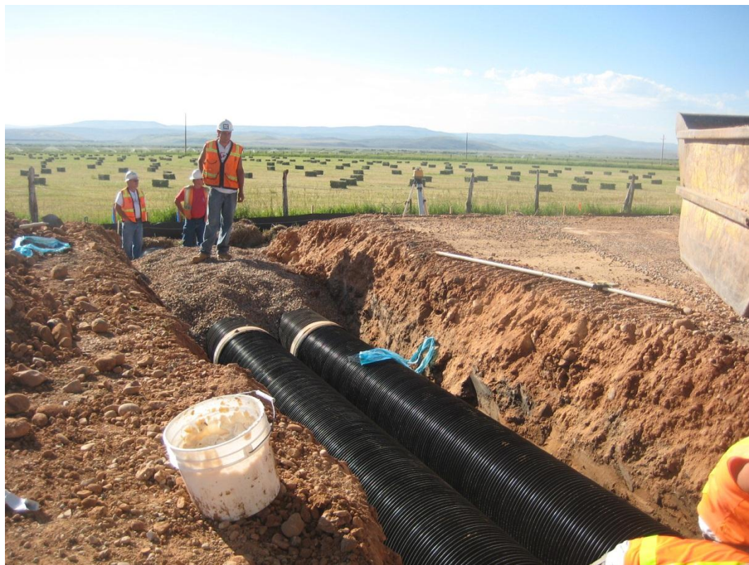
Figure 2. Photographs of the DuroMaxx pipe installation (photos from UDOT).
