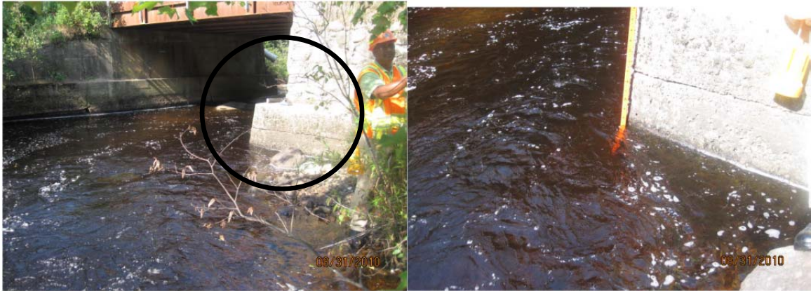
Figure 3-7: Photographs Showing Substructures of Bridge 2205690 Protruding into the Channel.
