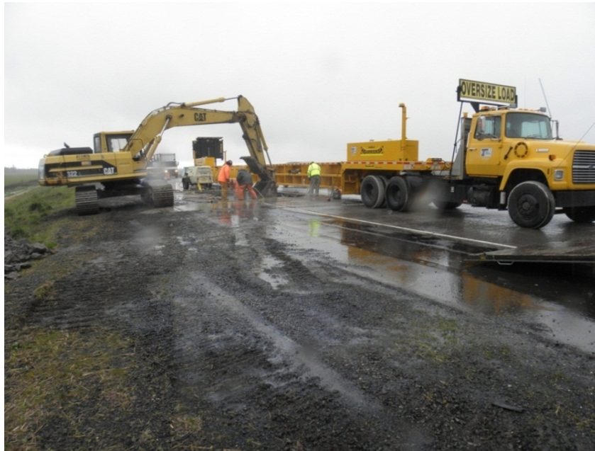
Figure 3.6: Workers Removing Concrete Pavement (Case Study #2)
