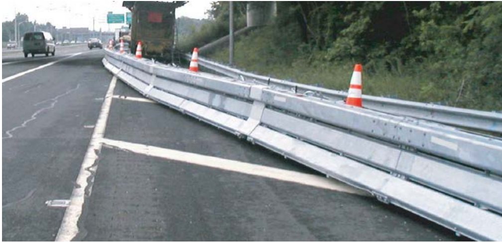
Figure 2.4: Armor Guard Barrier ( Barrier System 2008 )
