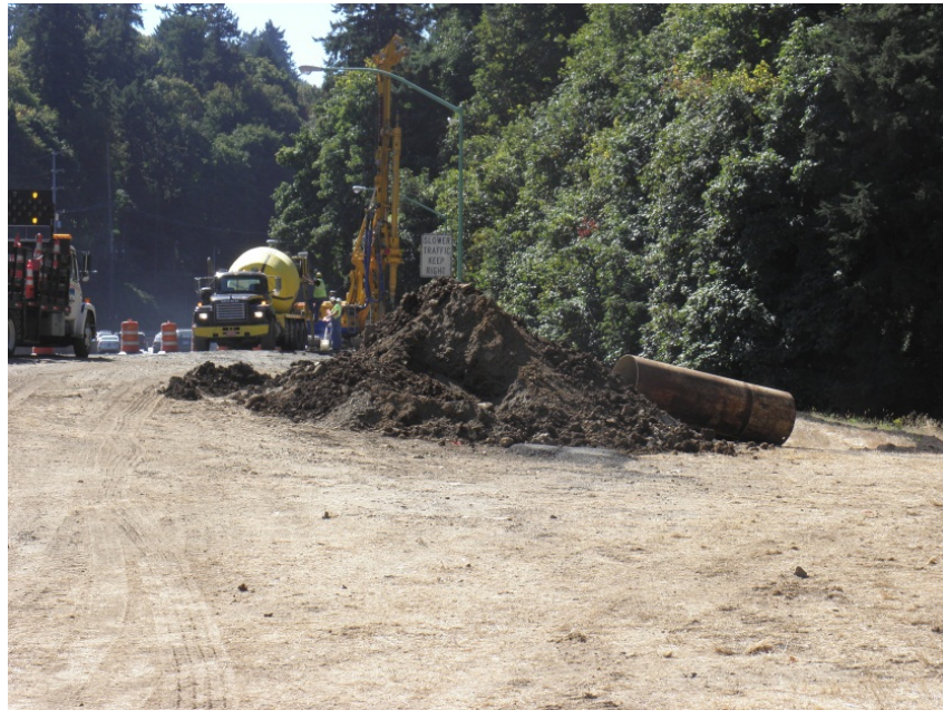
Figure 3.13: Worksite, September 11 (Case Study #4)
