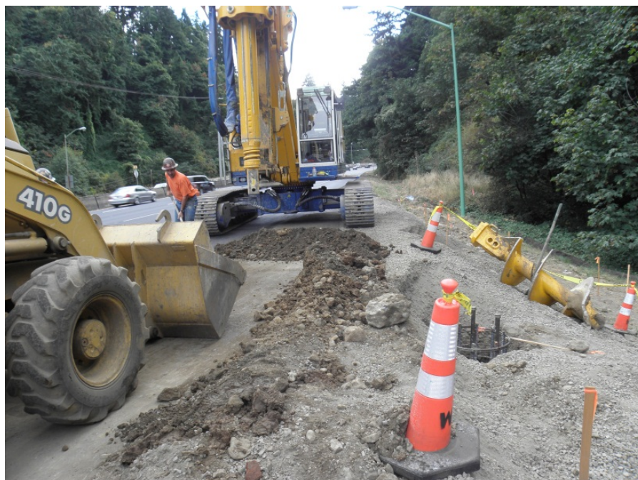
Figure 3.12: Workers Working on the Site, September 10 (Case Study #4)
