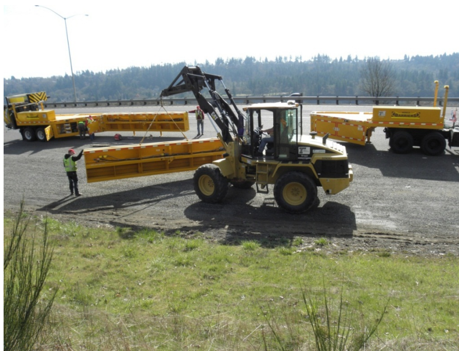
Figure 3.5: Adding a 20-foot Extension on the MBT-1® (Case Study #2)
