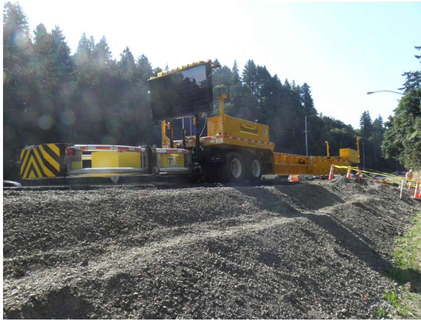
Figure 3.14: MBT-1® Parked Next to Drill Shaft
