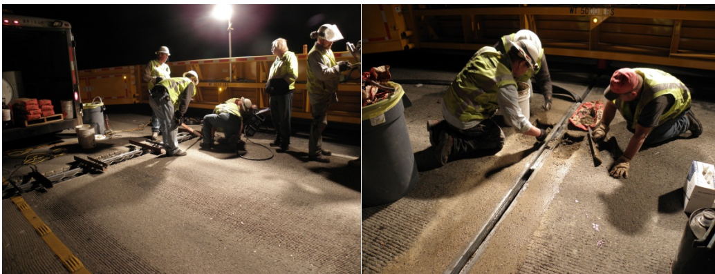
Figure 3.22: Workers Placing Joint (left); Workers Removing Concrete (right) (Case Study #6)
