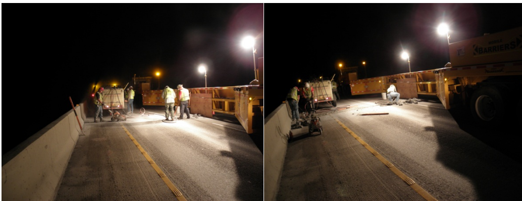
Figure 3.21: Workers Cutting Concrete (left); Workers Jackhammering Concrete (right) (Case Study #6)
