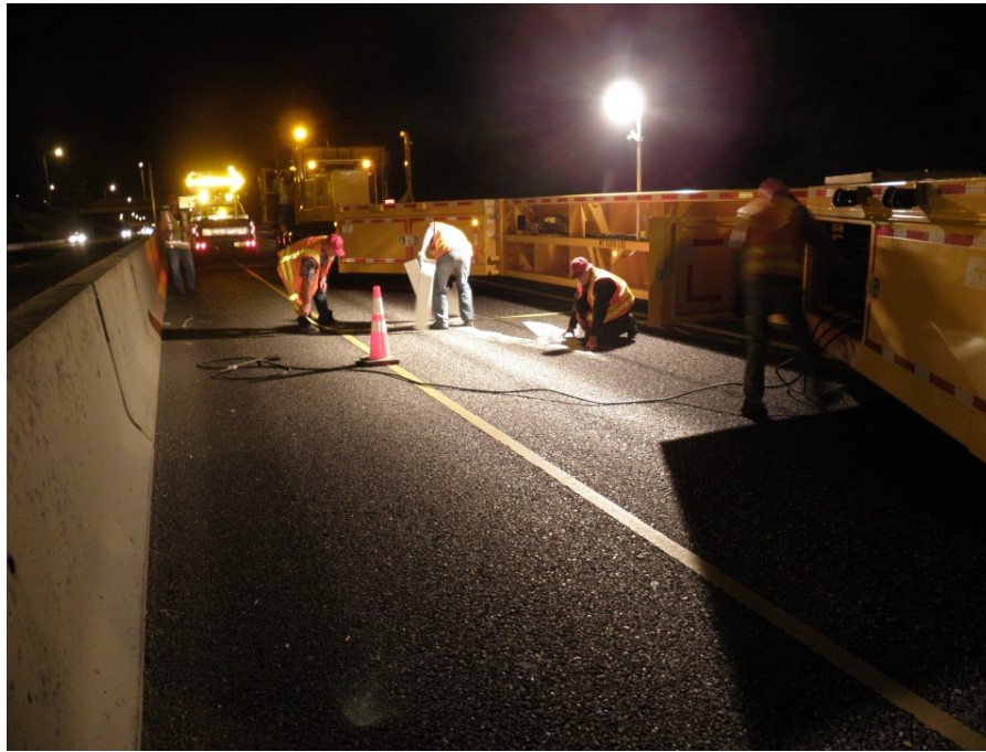
Figure 3.15: Installation of HOV Markers on I-5 Northbound (Case Study #5)
