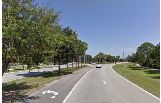
The safety and aesthetic contributions of median landscapes must be balanced against unobstructed views for drivers.
