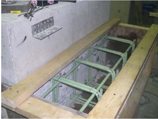
(a) Reinforcement inside a wooden form
