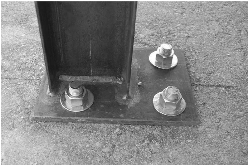
Figure 10. Pre-test Installation Photographs
