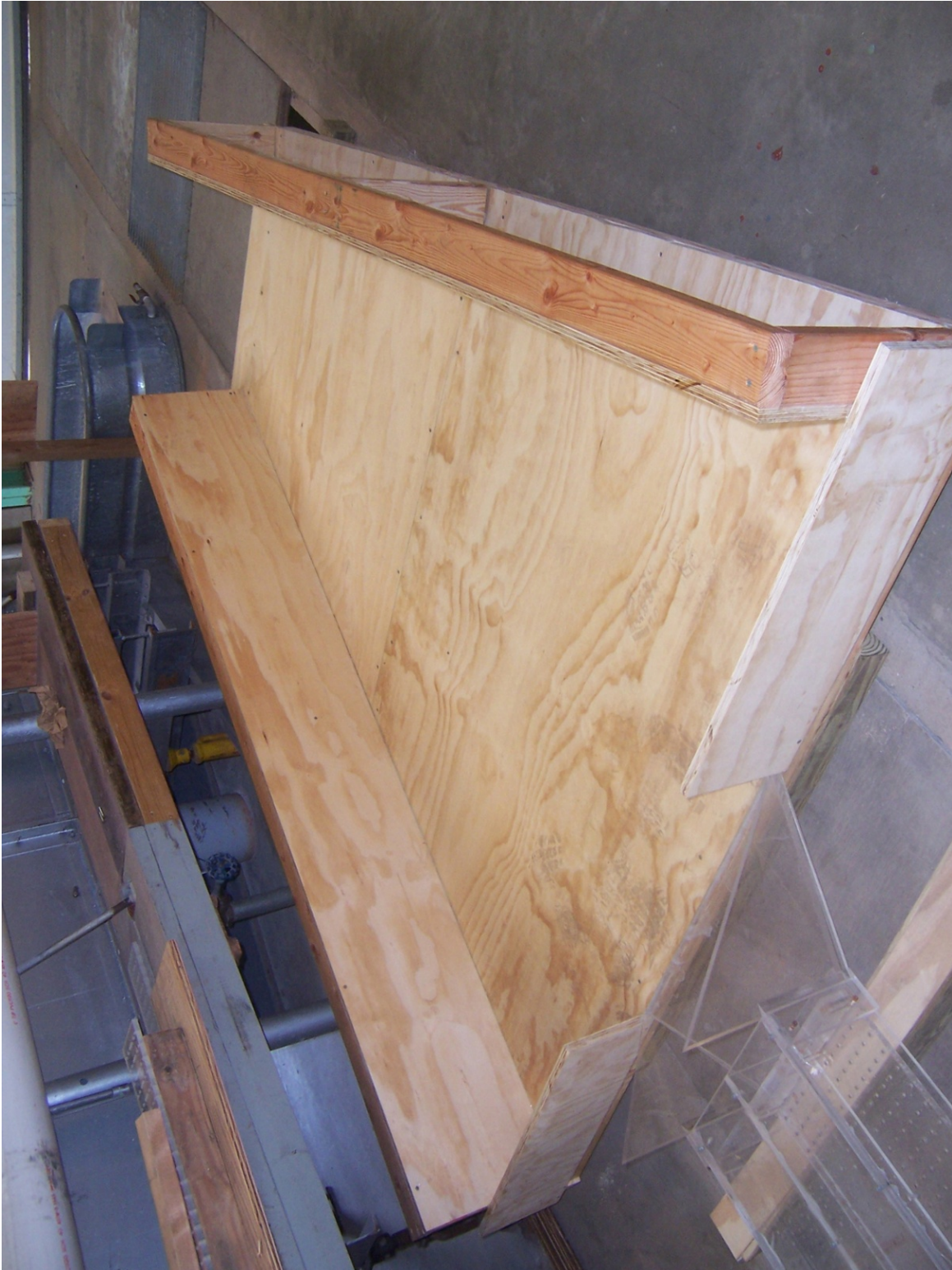
Figure 11. Downstream plywood channel after wingwall.
