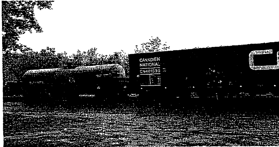
Figure 3.11 Buffalo/Cheektowaga Railyard Simulated Tank Leak
