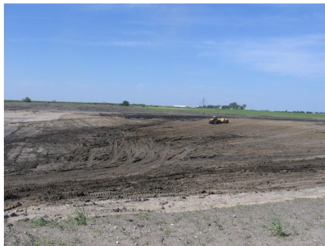
Figure 7. New construction site for US-20 in Calhoun County
