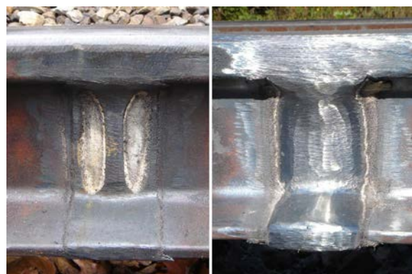
Figure 1. WGWs—Railtech Boutet (left); Orgo-Thermit (right)
