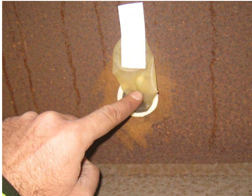
Figure 30. CHLOR*TEST sleeve adhered to surface and being massaged during extraction.
