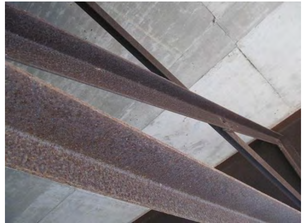
Figure 4. Typical cross frame condition near south abutment. Index = 3.
