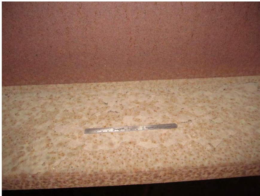
Figure 21. Poulitice corrosion on an interior girder flange in downtown Des Moines. This is typical of conditions observed on the tops of many interior horizontal elements. Close examination and testing confirms this chalky film is primarily a mixture of dirt and salts.
