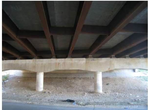
Figure 4. Interior girders of westbound mainline bridge showing good patina performance.
