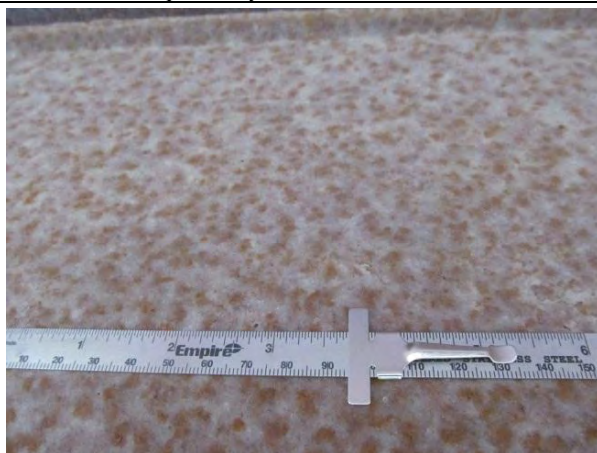
Figure 5. Poultrice on flange before washing.
