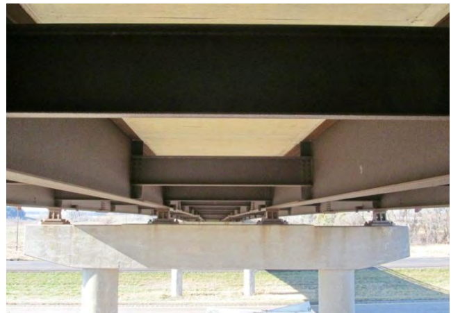
Figure 4. East pier viewed from east abutment. Drainage deflectors separating spans effectively.
