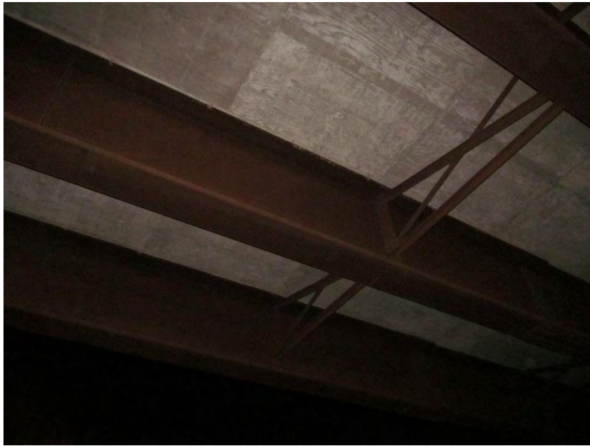
Figure 1. Girder and cross-frames near mid-span; representative of conditions throughout the structure.
