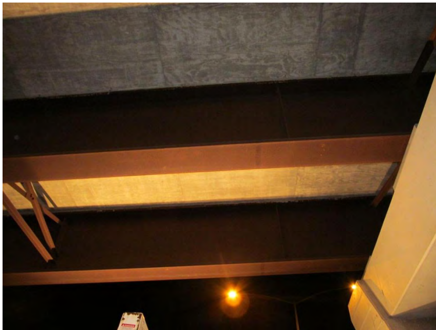
Figure 2. Girders and cross-frames near the intermediate pier.
