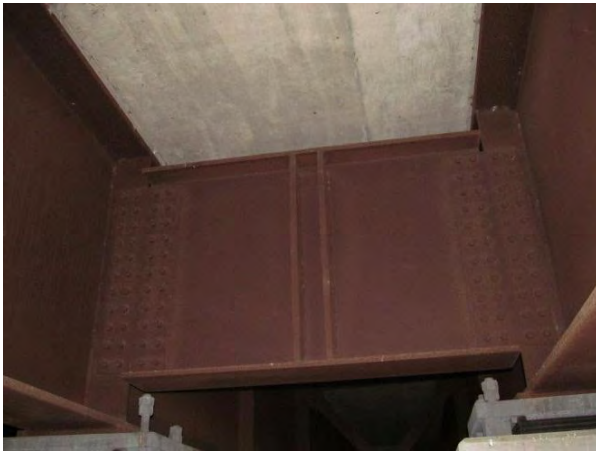
Figure 3. Stiffened I-beam diaphragm at pier.
