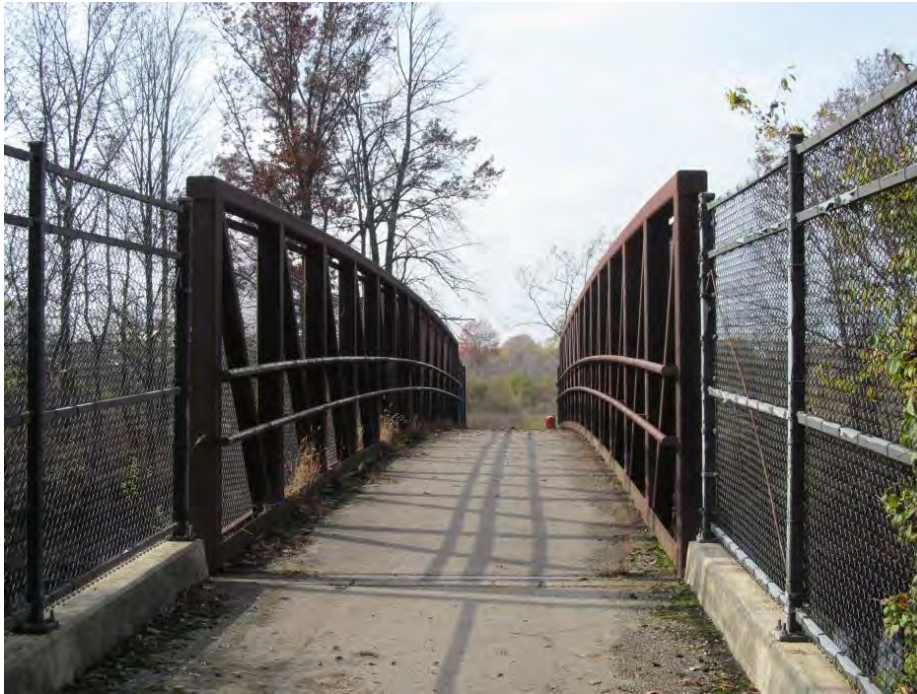
Figure 6. Pedestrian bridge carrying a trail over the Des Plaines River in an Illinois forest preserve, with no apparent salt exposure.
