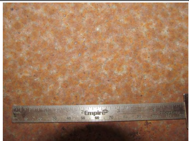
Figure 6. Flange poultrice partially reduced by washing.
