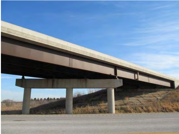
Figure 1. Overall appearance of north end of bridge showing high skew.
