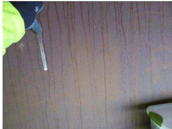
Figure 5. Interior web performing well.
