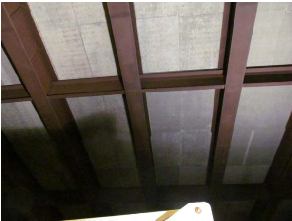
Figure 3. Middle of south span.
