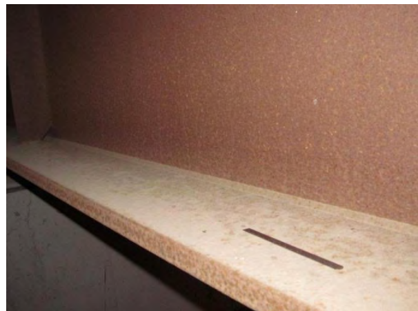
Figure 6. Interior girder bottom flange with heavy poultrice corrosion viewed from arm's length.
