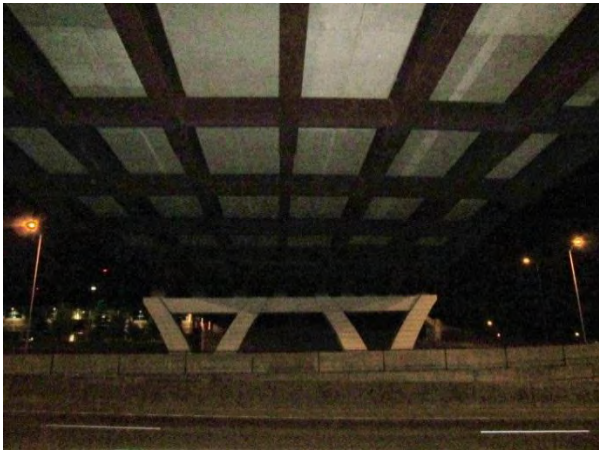
Figure 1. Overall view toward north two spans and north pier.
