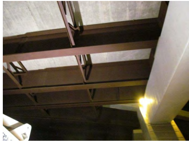
Figure 2. West half of girders near pier, where ramp comes in (background).
