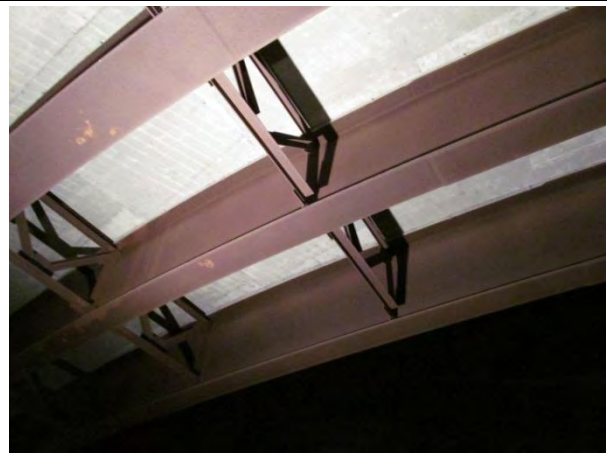
Figure 6. Some localized discoloration and flaky areas on otherwise good patinas near pier.
