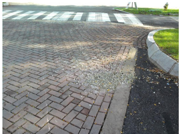
Figure 17: Run on from intersecting MUB drive.
