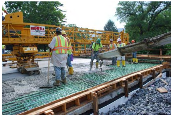
Figure 12. Concrete being vibrated
