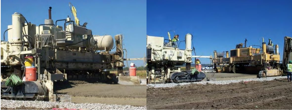
Figures 8 and 9. Concrete passing through the paver
