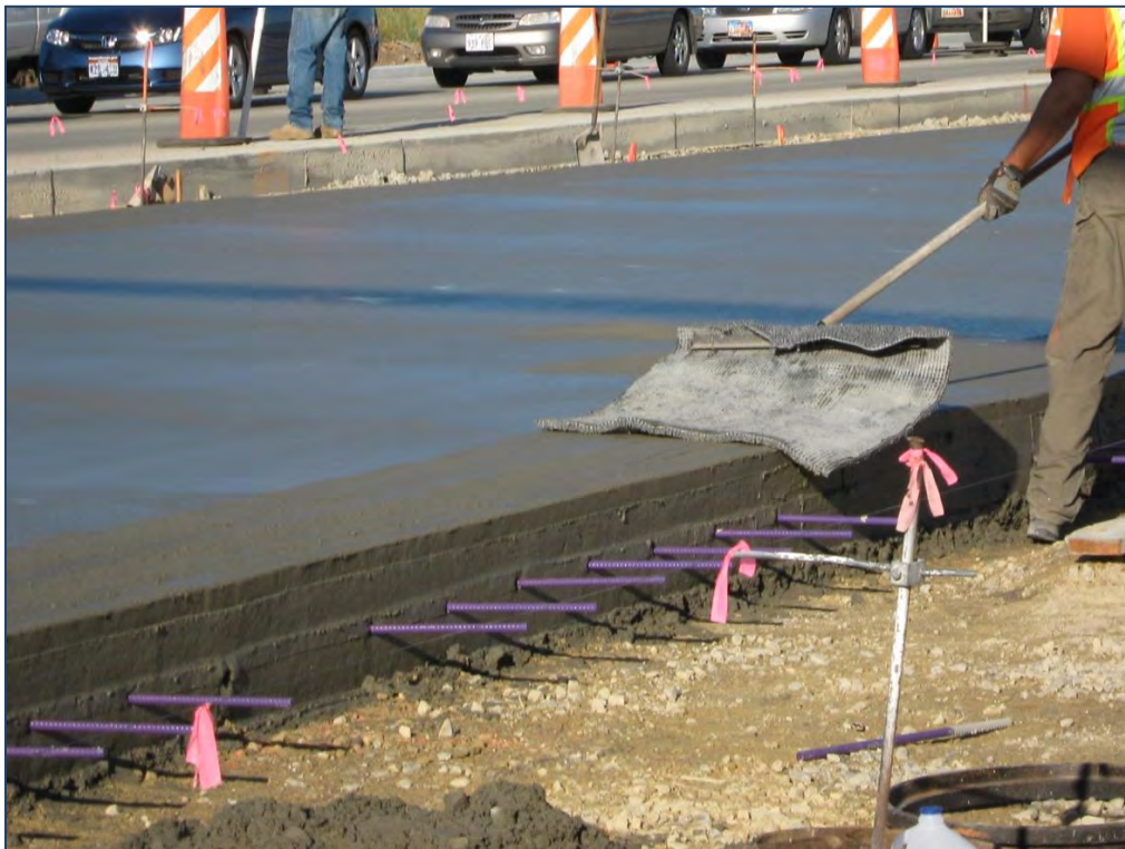
Figure 4. Ternary mixture maintained edges and finished well
