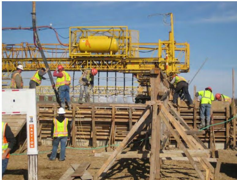
Figure 10. Concrete being placed and vibrated
