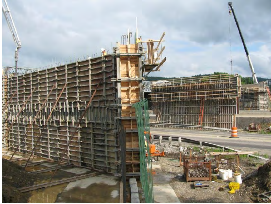
Figure 1. I-86 Coopers Plains bridge abutment stem structure, New York
