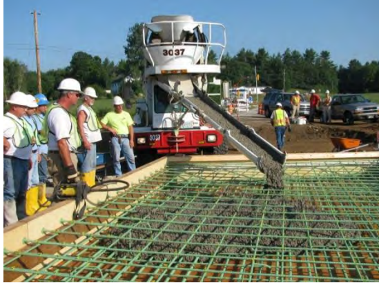
Figure 7. Bridge deck with concrete being placed
