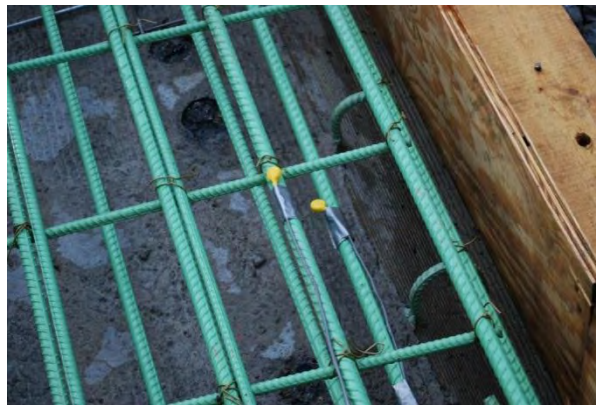
Figure 11. Two i-buttons being embedded on site
