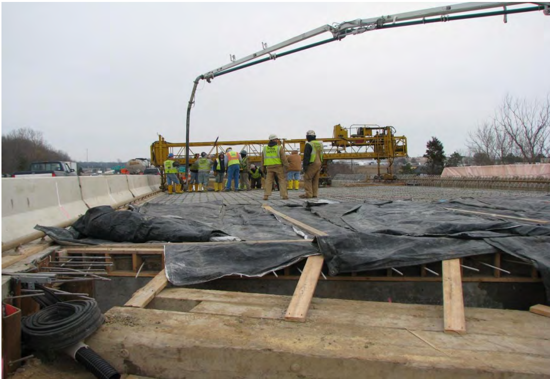
Figure 1. I-94 Riverside drive bridge deck placement
