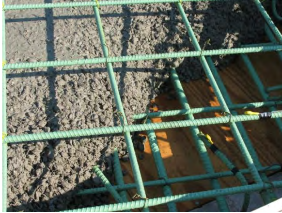
Figure 10. Two i-buttons being placed
