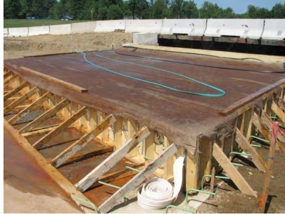
Figure 13. Concrete being cured with burlap
