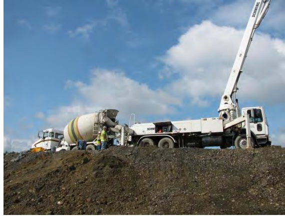
Figure 6. Concrete being pumped
