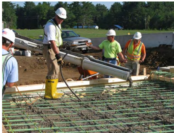
Figure 8. Concrete being vibrated
