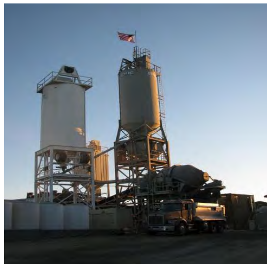
Figure 4. Central mix plant
