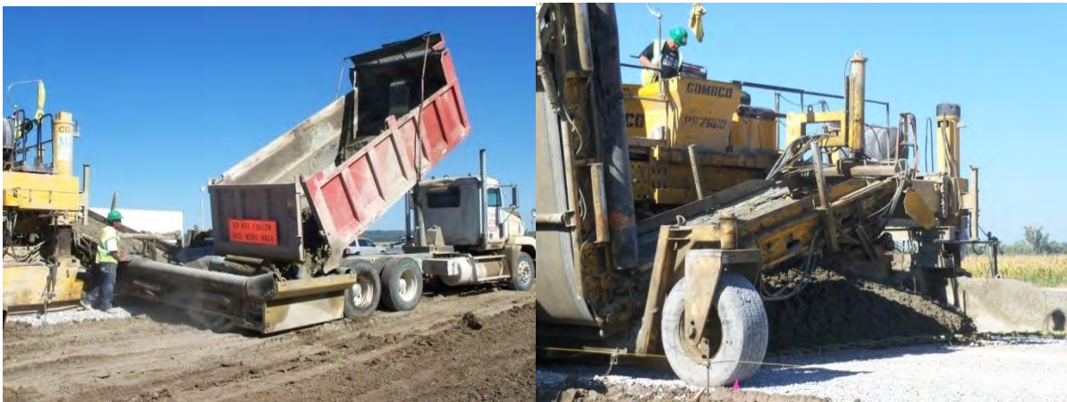
Figures 6 and 7. Concrete being dumped into a belt placer and spread by the placer
