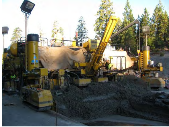
Figure 8. Concrete passing through the paver
