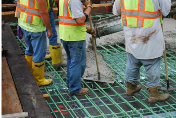
Figure 7. Concrete being spread by construction crews
