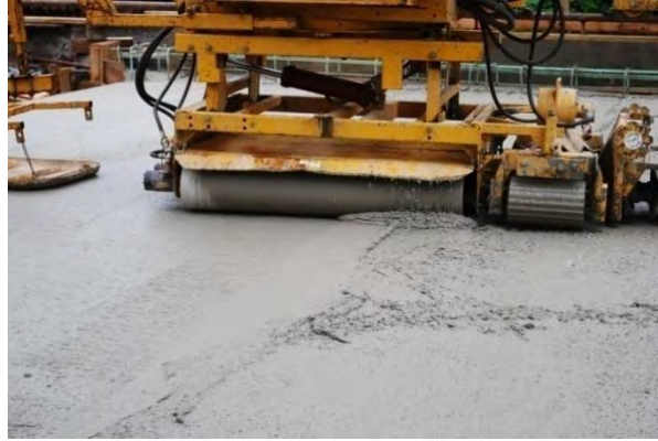
Figure 10. Concrete being finished
