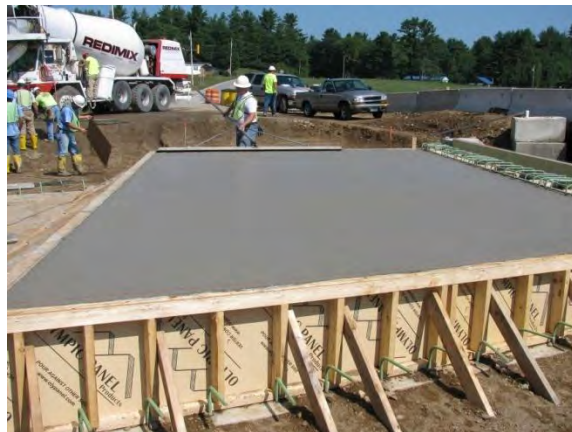
Figure 12. Concrete being finished
