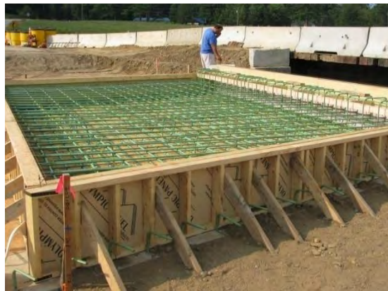
Figure 6. Bridge deck with removable wood form
