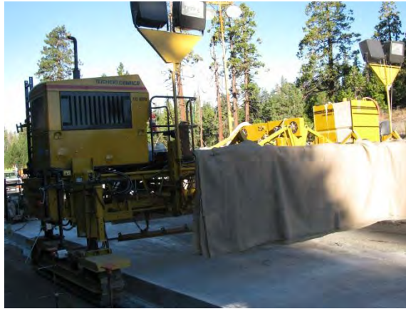
Figure 12. Texturing/curing machine
