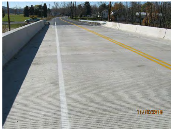
Figure 14. Bridge deck surface four months after construction
