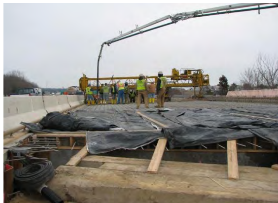
Figure 11. Curing blankets for concrete curing
