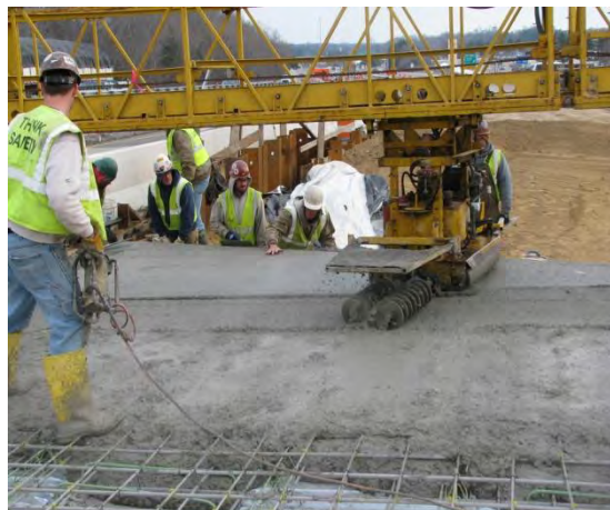
Figure 8. Concrete being placed
