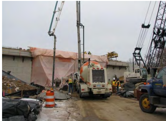
Figure 10. Concrete heated tent enclosure below the deck
