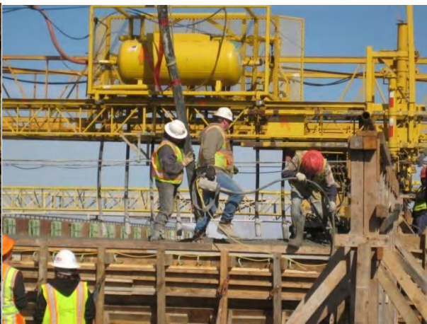
Figure 7. Construction crew placing concrete, pouring and vibrating
