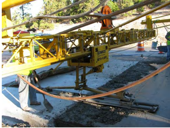
Figure 11. Concrete surface being sealed by Auto-Float
