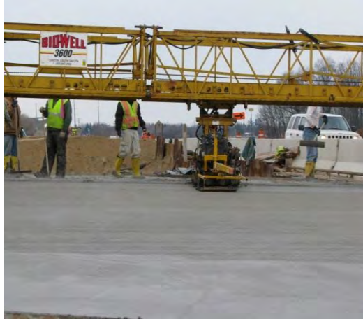
Figure 9. Concrete being finished
