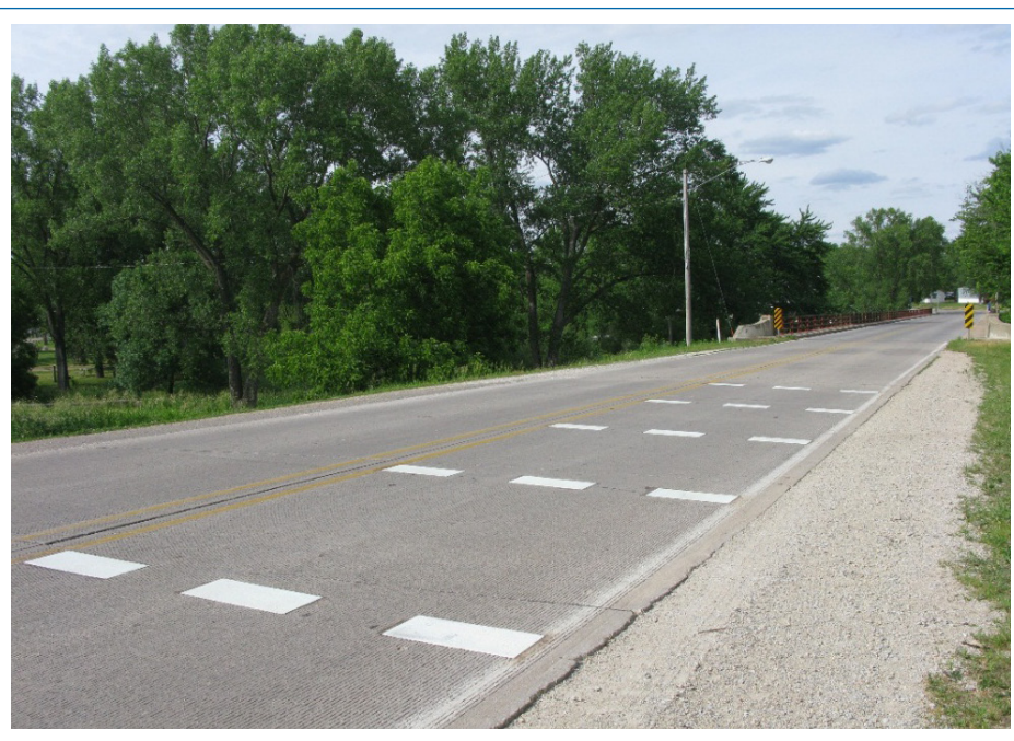
Transverse treatment at Quasqueton south entrance
