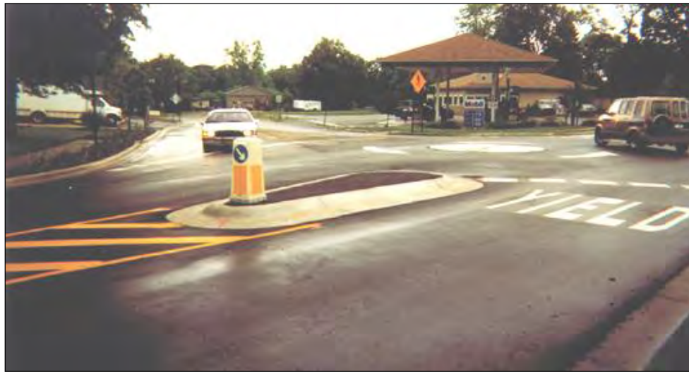
Figure 7: Mini-roundabout in Michigan (Waddell and Albertson, 2005)
