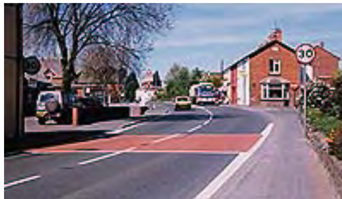
Figure 45: Treatment used in Shropshire, UK (DETR, 2005)
