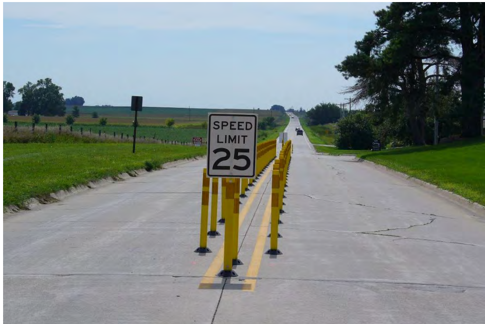
Figure 21: Creation of a center island with channelizers
