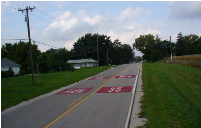
Figure 44: Colored pavement markings in Dexter, Iowa
