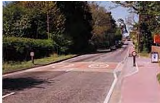
Figure 42: Pavement markings used as entrance treatment (DETR, 2005)
