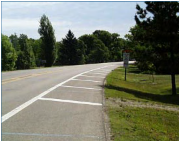
Figure 25: Lane narrowing with transverse shoulder stripes
