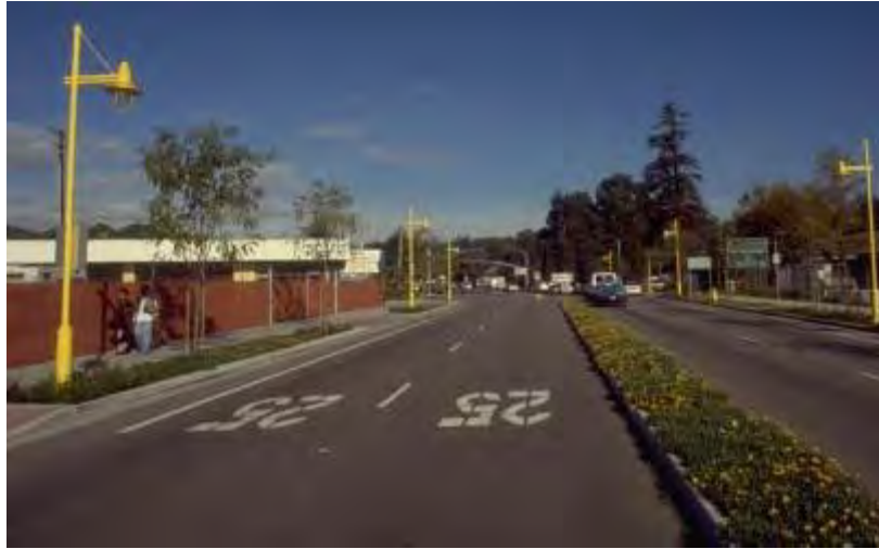
Figure 47: Speed limit pavement markings (CWS, 2003)
