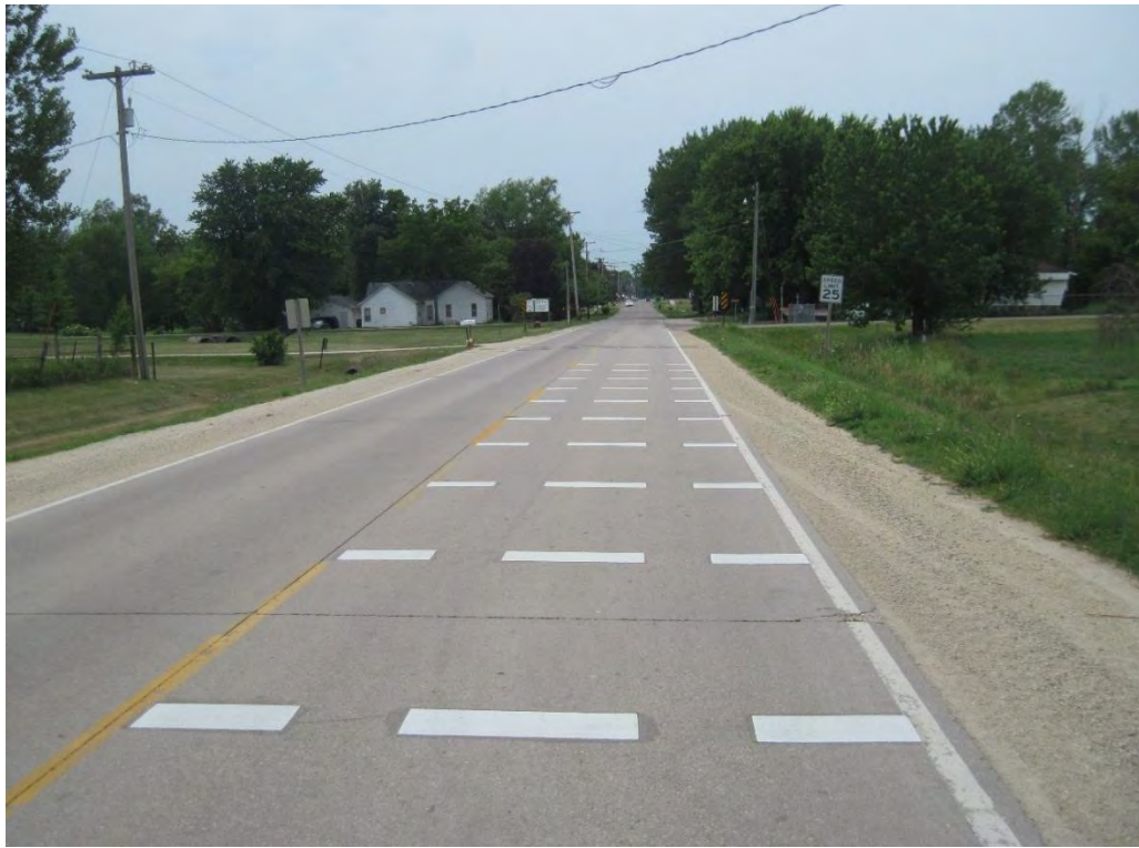
Figure 40: Transverse bar treatments
