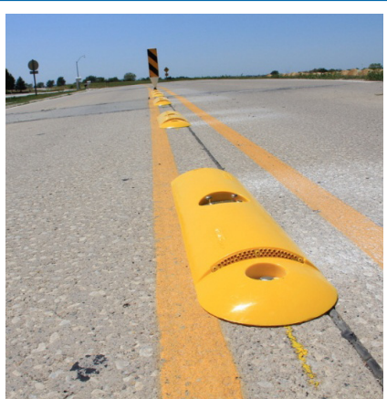
Close-up of mountable curbing
