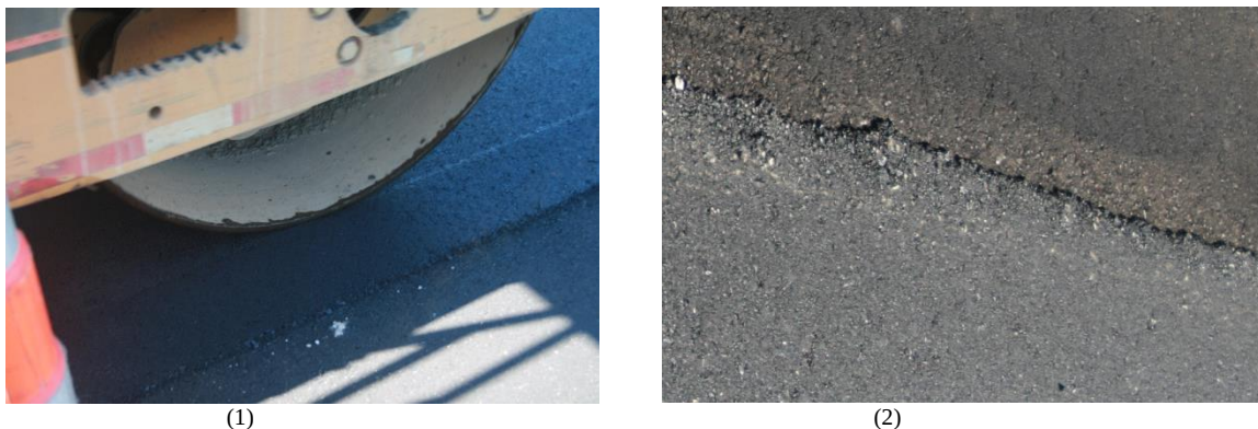
Figure 2. Butt joint construction with hot pinch (pictured on US 61)
