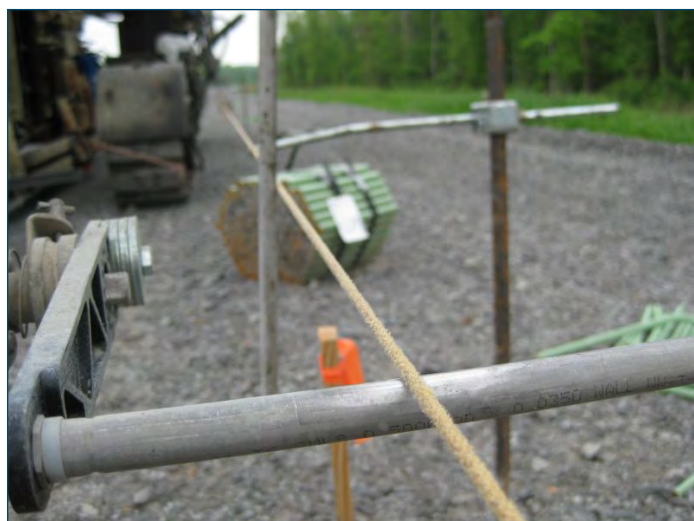
Figure 37. Sensor rods that track alignment and elevation
