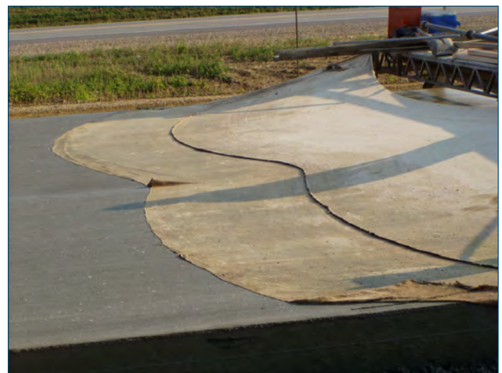
Figure 54. Burlap drag attached to a work bridge
