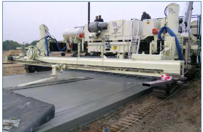
Figure 44. Automatic longitudinal float attached to the back of a paver
