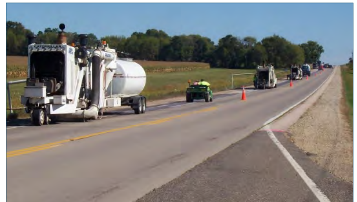
Figure 59. A grinding large-scale concrete pavement resurfacing operation
