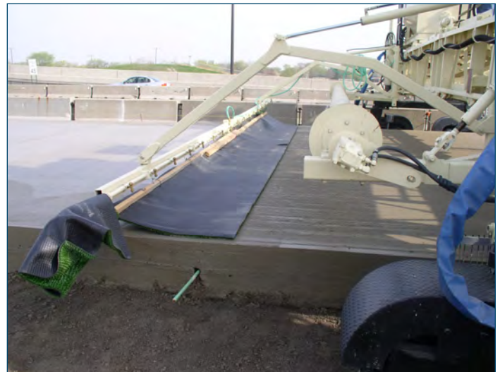
Figure 53. Turf drag attachment on a texture machine
