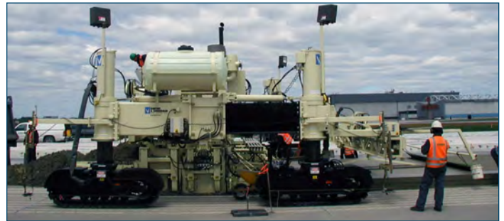
Figure 38. Side forms should be parallel to the stringline
