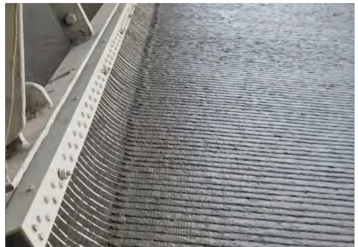
Figure 7. Longitudinal tining of a newly placed concrete surface
