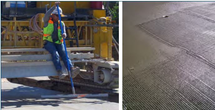
Figure 17. Manual longitudinal tining leading to undesirable texture variability (photo courtesy of Jim Grove)
