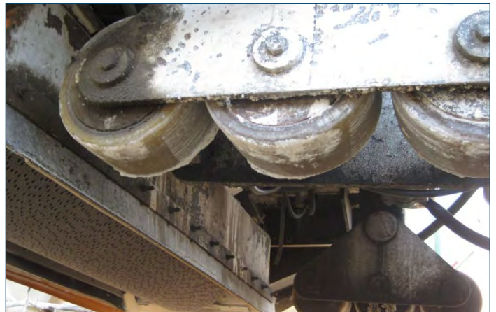
Figure 63. Bogie wheels supporting grinding head should be checked periodically
