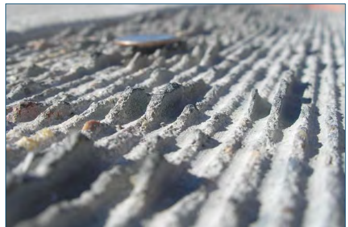
Figure 31. Concrete fins that can remain immediately after grinding operation
