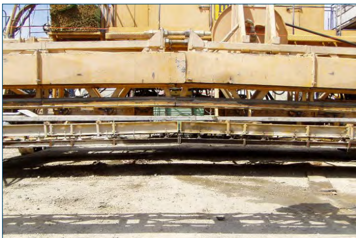
Figure 43. Forming pan set for a crowned pavement
