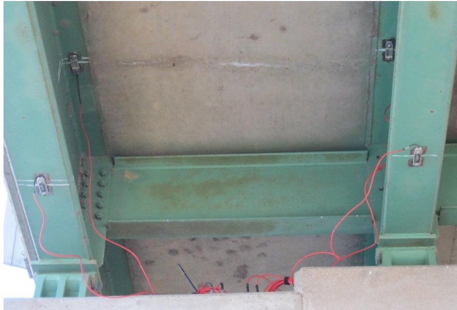
Figure 10. Sioux County Bridge instrumentation setup
