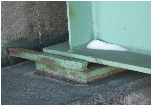
a. Abutment bearing
